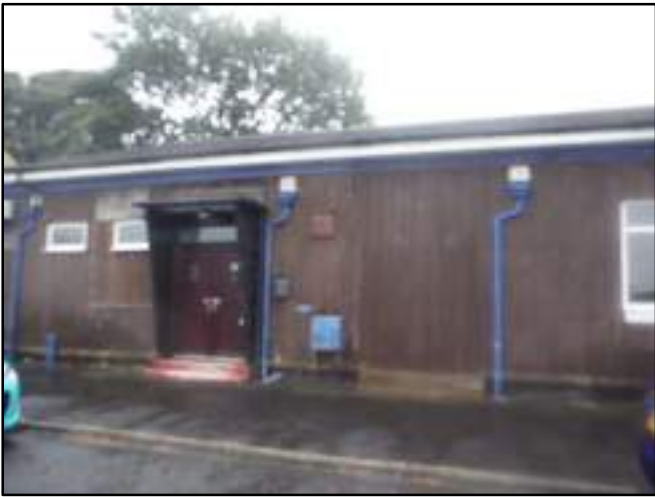
P1: Looking at west face of building from Towneley Road
