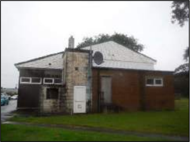
P3: Looking at southern face of the building
