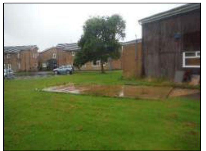
P6: Concrete slab in the south-east of the site
