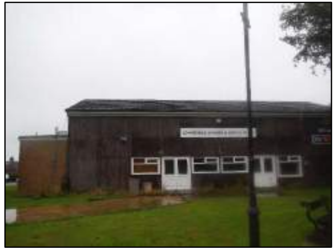
P2: Looking at east face of building from Bowling Green area
