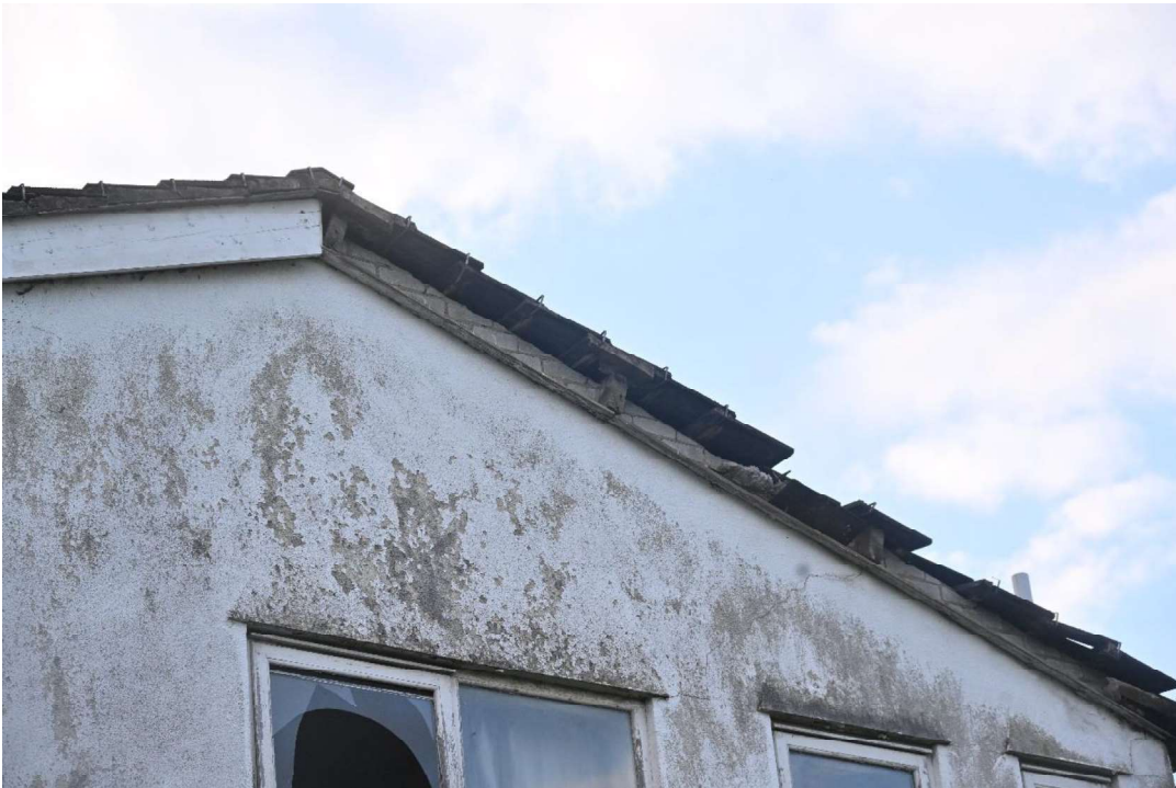
Image 4 Roof damage at rear of house
