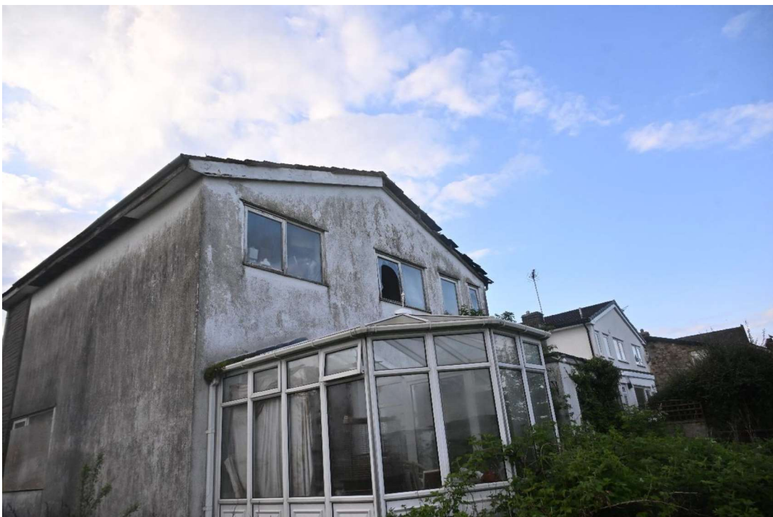
Image 2 Rear of house from garden with signs of damp and damage to soffits roof etc
