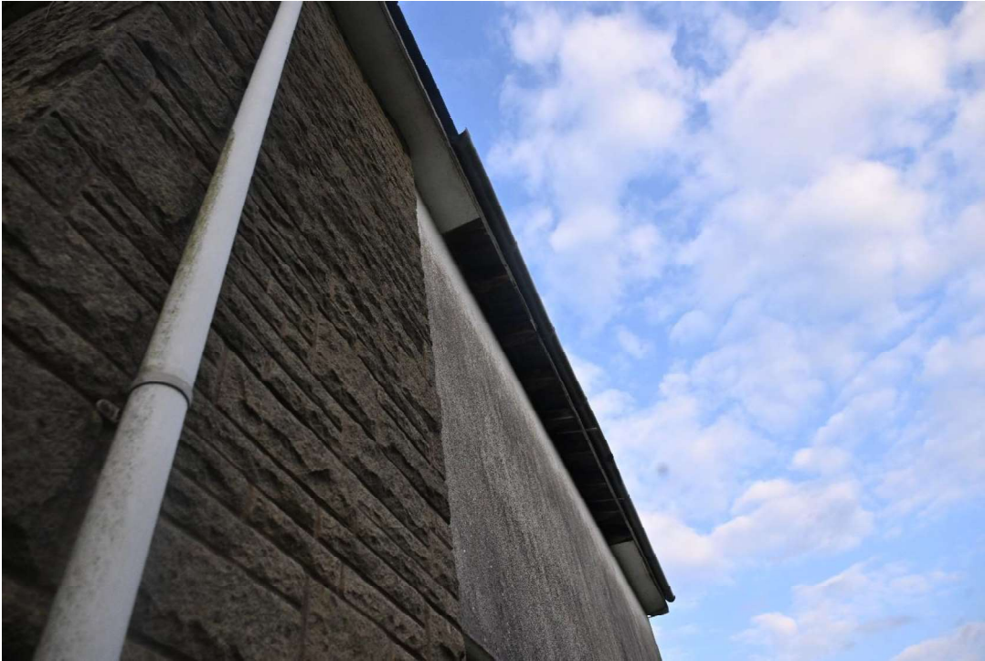
Image 3 Missing soffit boards where jackdaws are nesting
