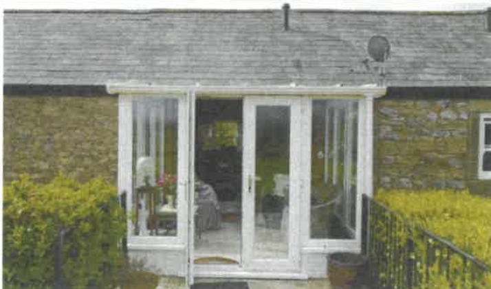
Rear Elevation of the conservatory
