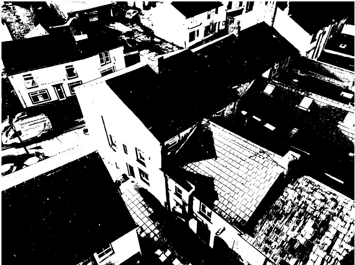
2 – The rear of the building, showing both roofs.
