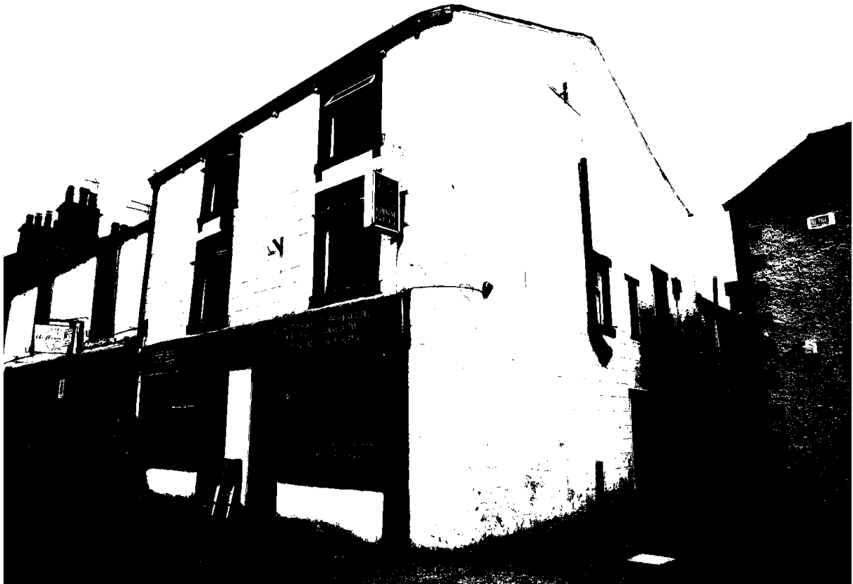
1 – The front and gable end of the building.
