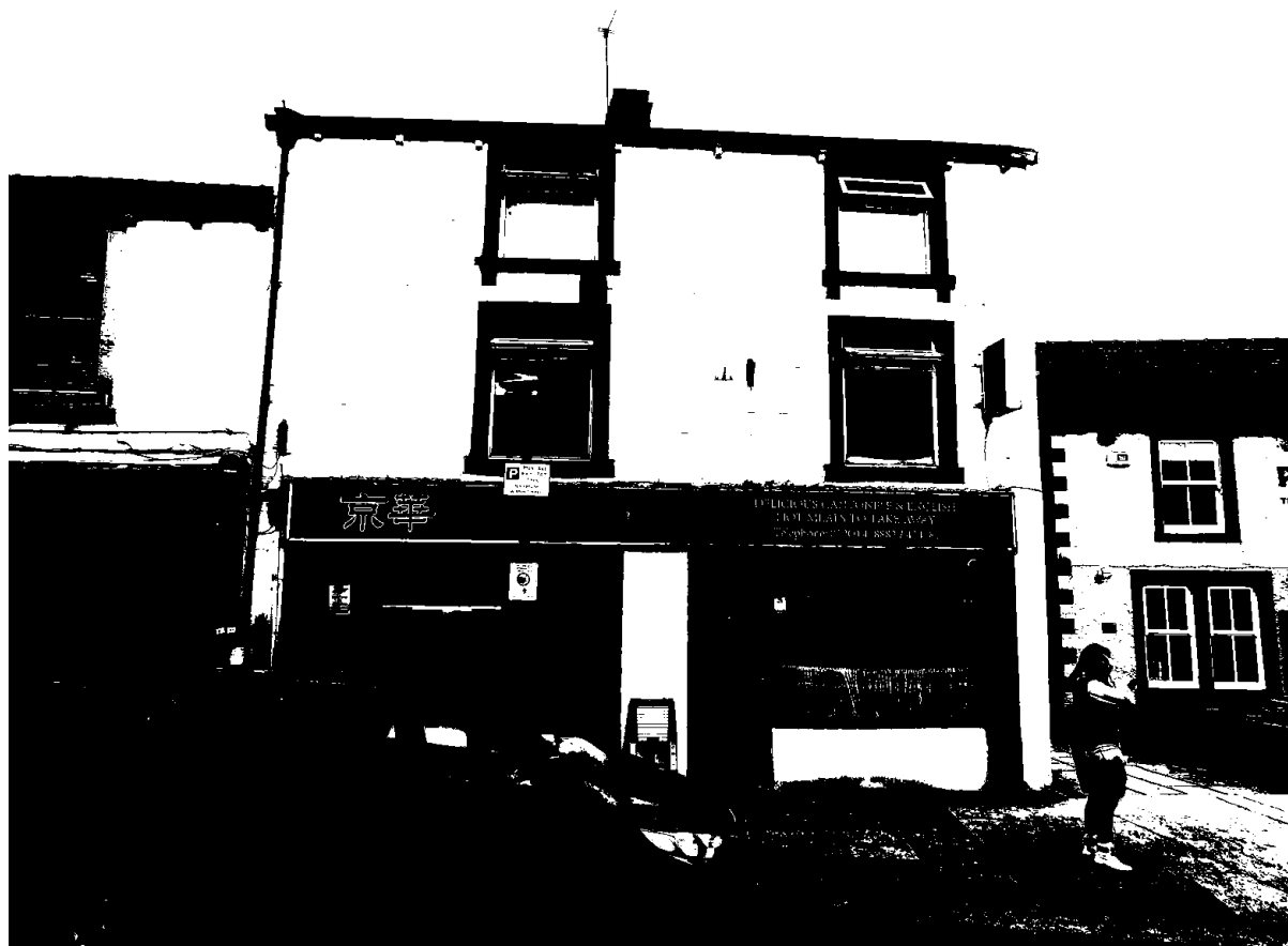
3.1a – The front of the building.
