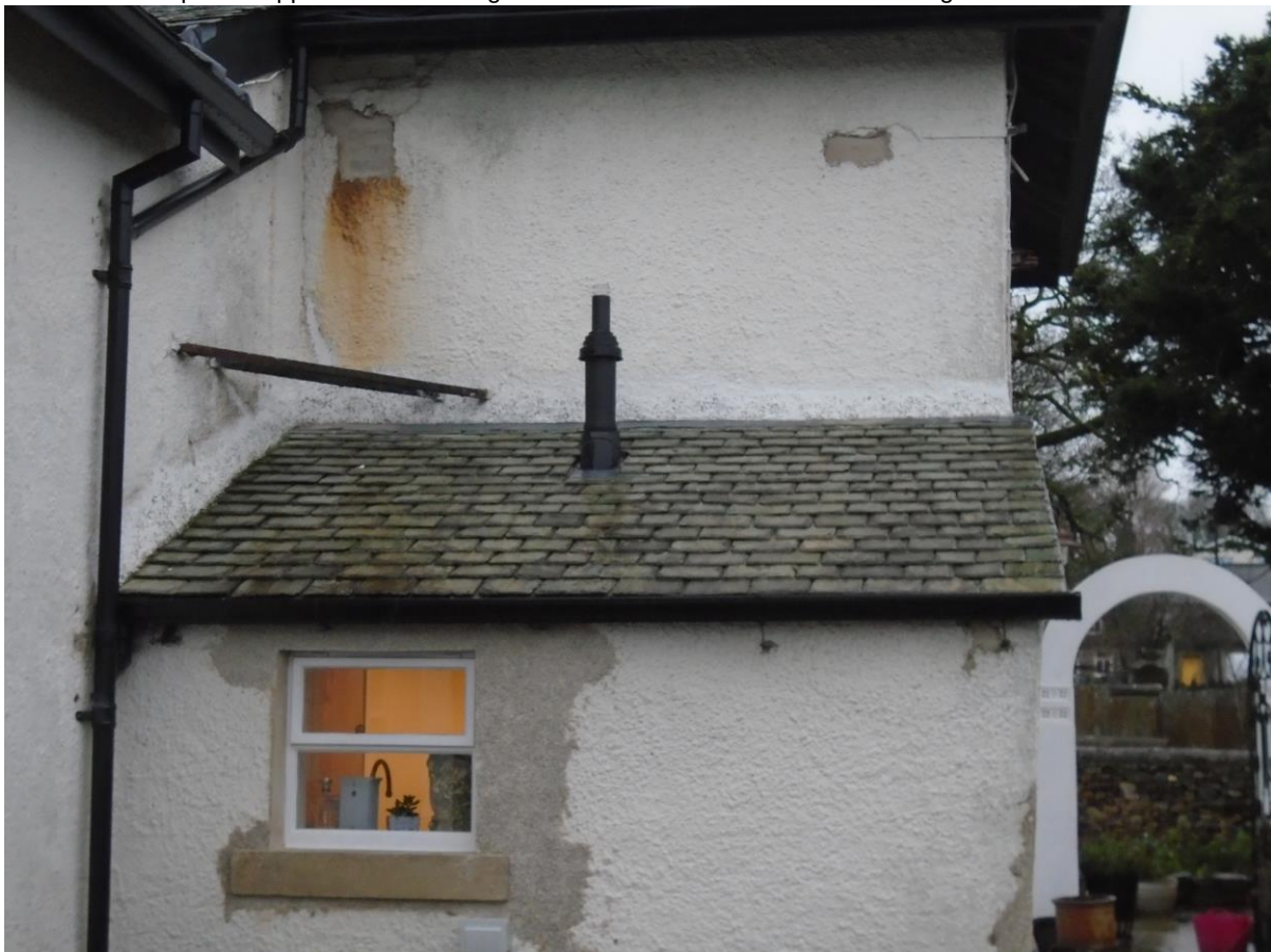
Lean to roof
