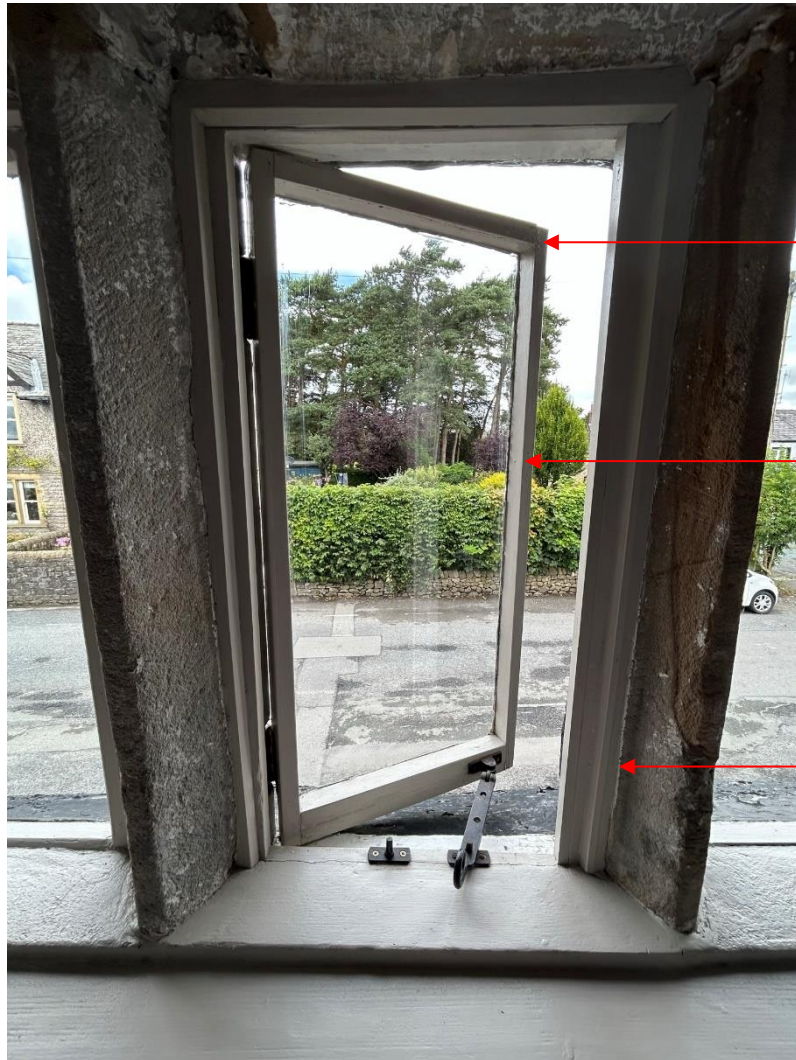
Photo 10: First floor side-hung casement (internal)
