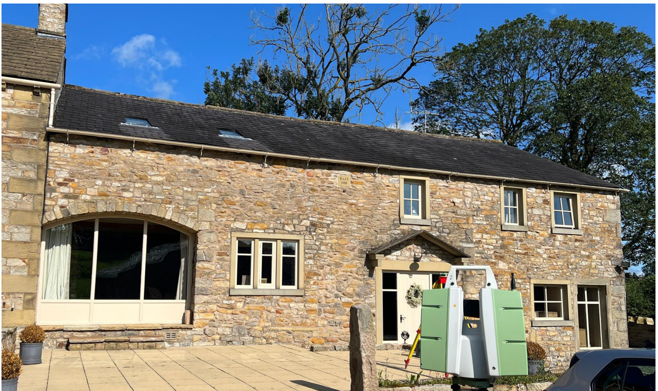
Figure 4) Barn part with former cart entry (the arched lintel of which appears to have been lowered) with some inserted openings (1988) and rooflights
