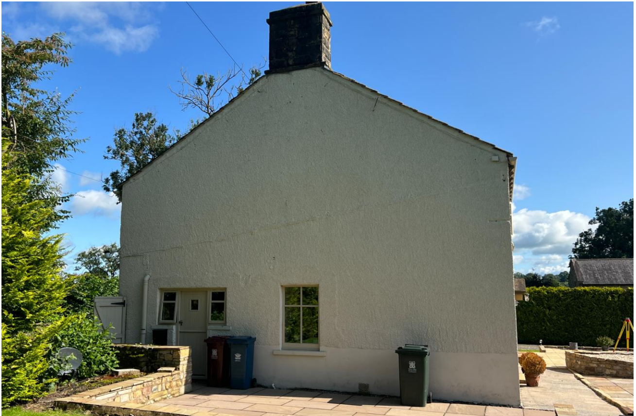
Figure 5) Western gable – both openings appear inserted (non-original)
