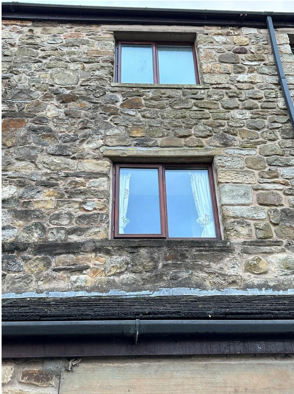
First and second floor windows on left hand side of front elevation
