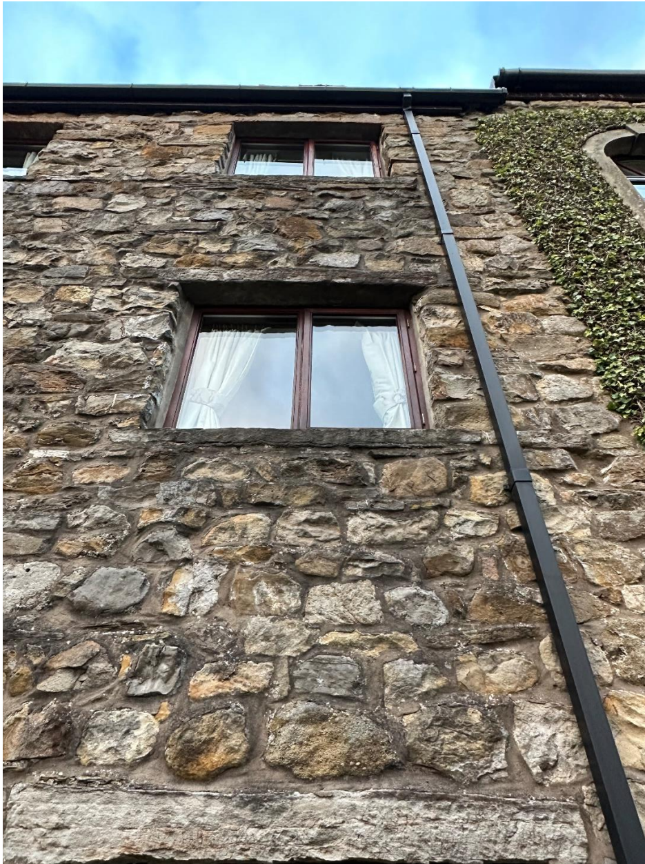
First and second floor windows on right hand side of rear elevation
