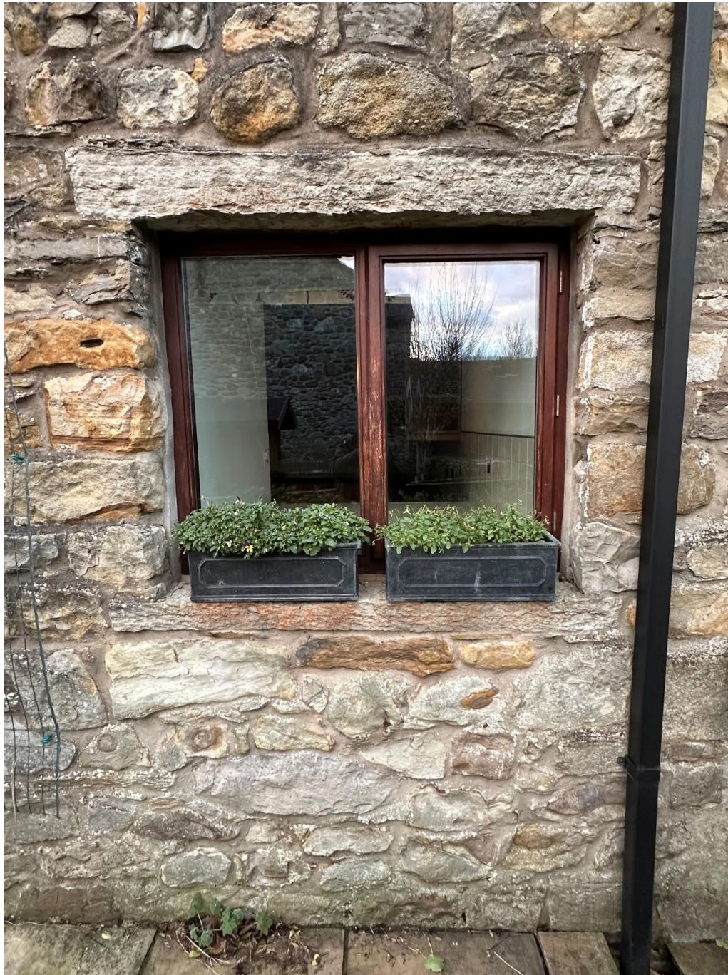
Right hand ground floor window on rear elevation
