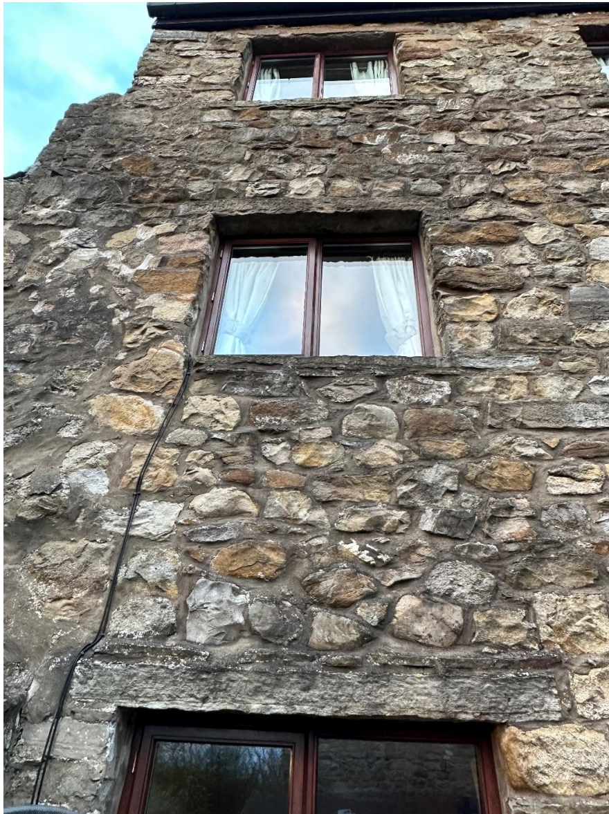
First and second floor windows on left hand side of rear elevation
