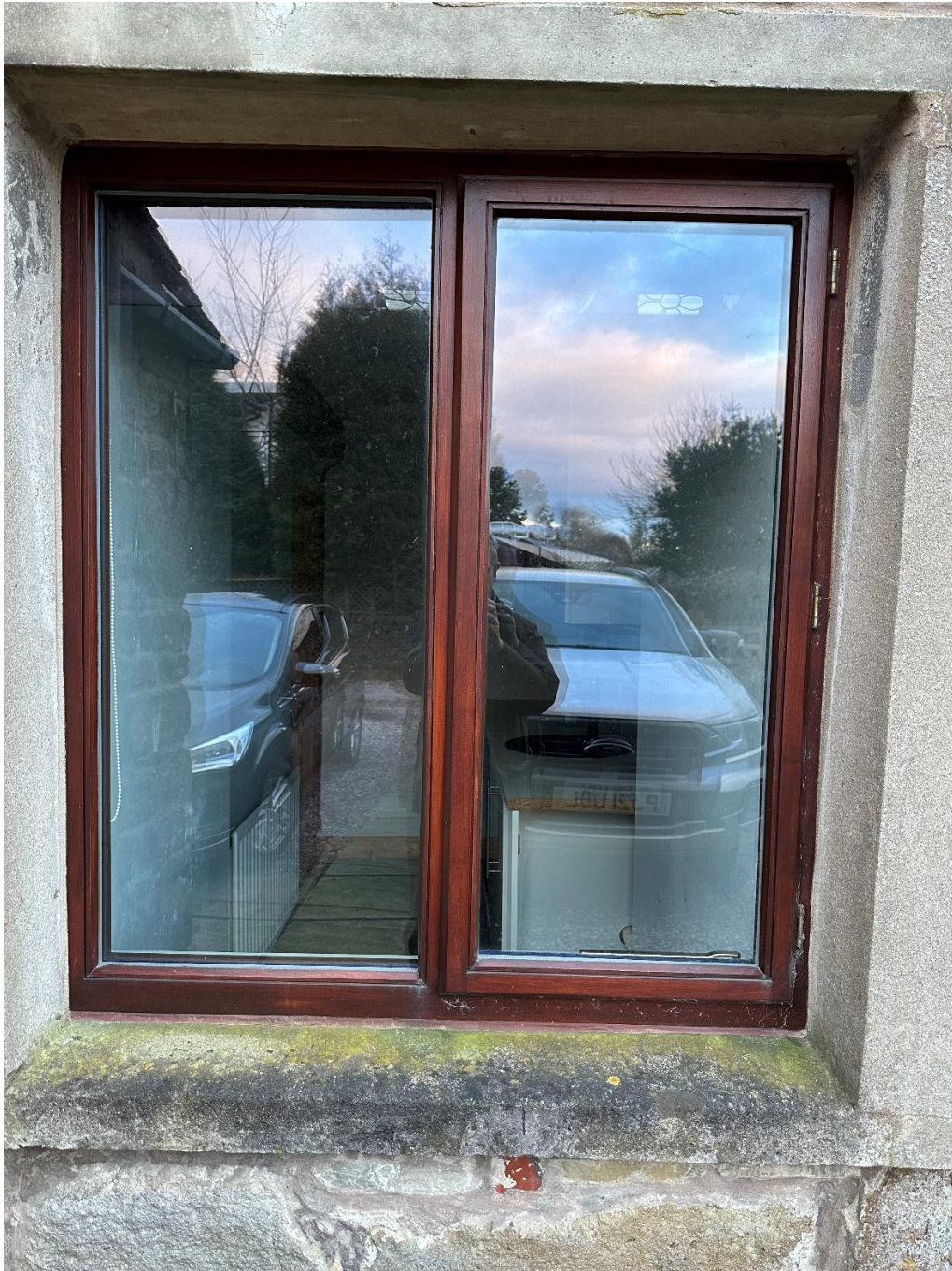
Close up photograph of front ground floor window on front elevation
