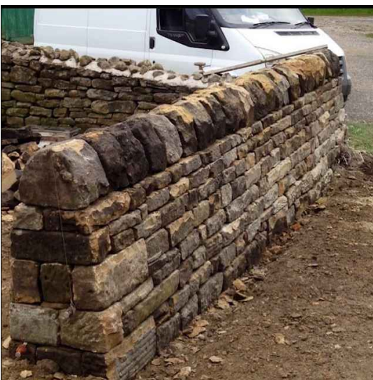
Stone boundary wall
