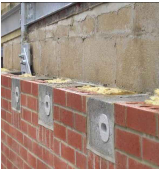
Bird box to be integrated into gable ends, suitable for a range of bird species
