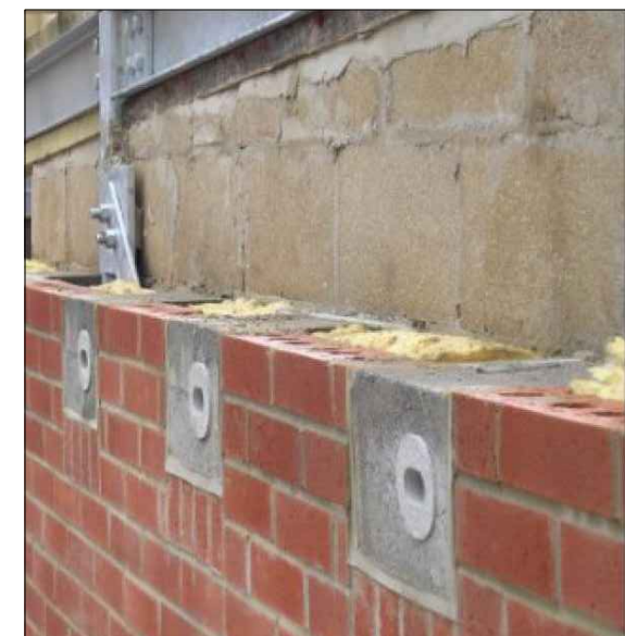
Bird box to be integrated into gable ends, suitable for a range of bird species
