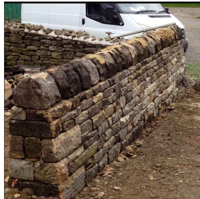
Stone boundary wall.
