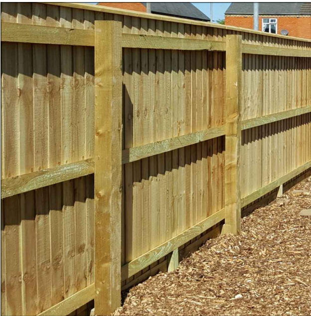
Feather board fencing between dwellings. Refer to drawing ref: 1035-103 for full details
