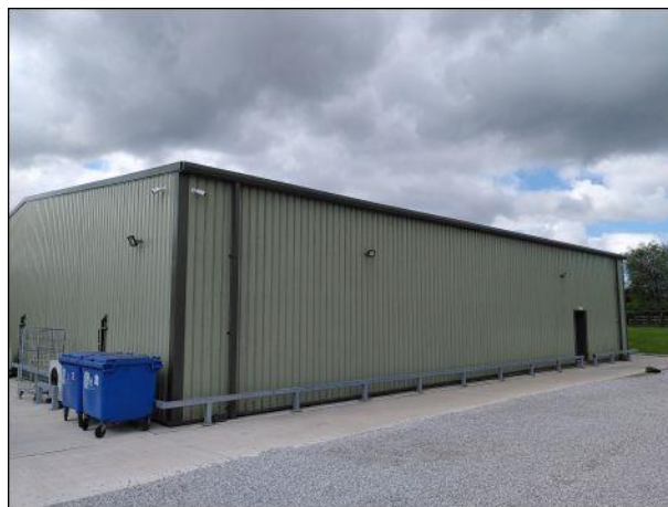
Photo 10: Building 1, northern elevation
