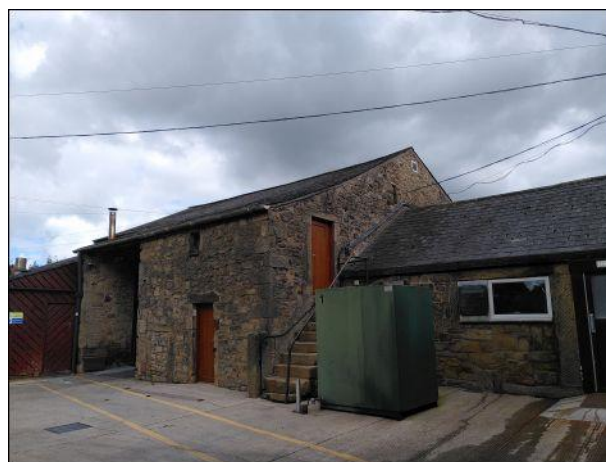
Photo 18: Building 2, southern elevation, eastern end
