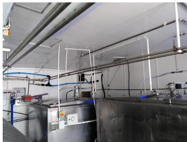
Photo 20: Internal area of Building 2
