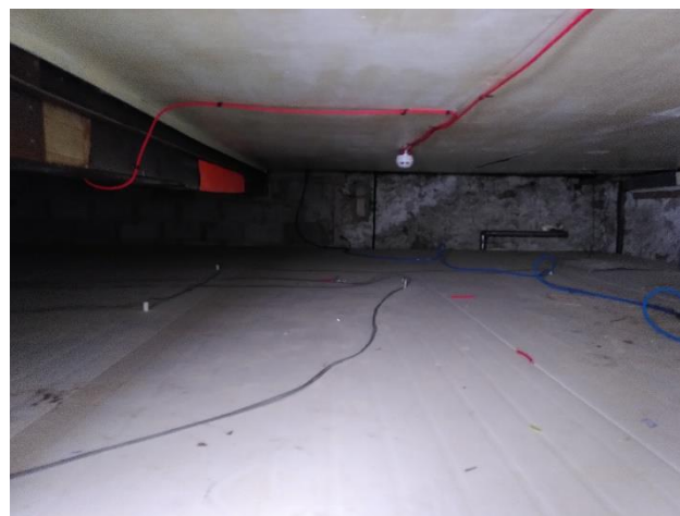
Photo 22: Void between working area and ceiling, Building 2
