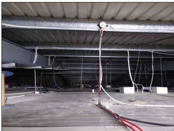
Photo 15: Building 1, internal area, southern end
