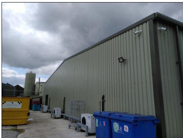
Photo 9: Building 1, eastern elevation
