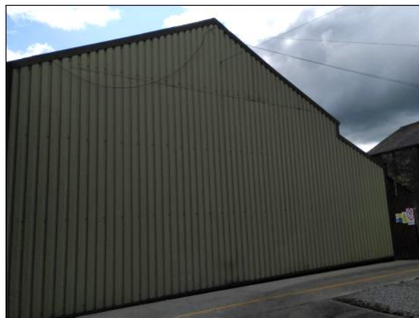
Photo 16: Building 2, western elevation
