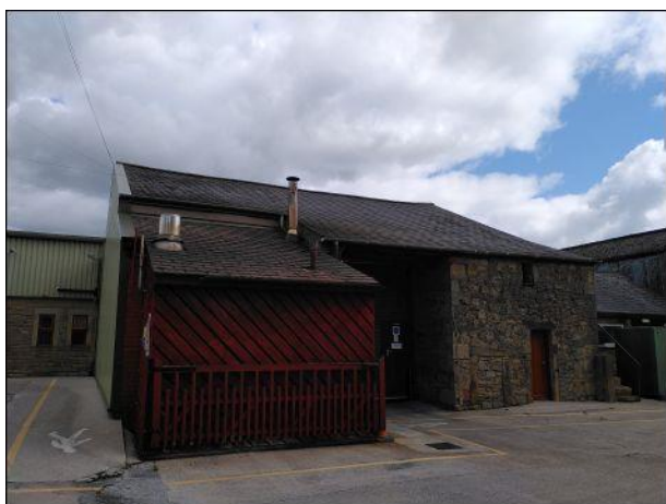
Photo 17: Building 2, southern elevation, western end
