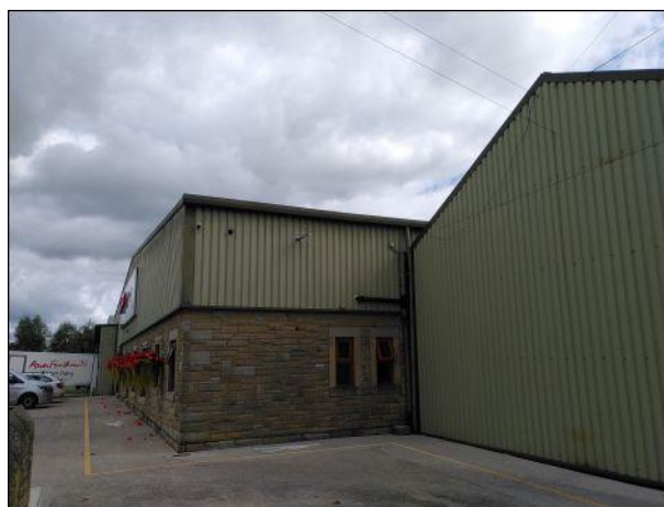
Photo 12: Building 1, western elevation, southern end
