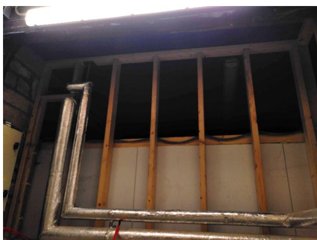
Photo 21: Roof void at Building 2
