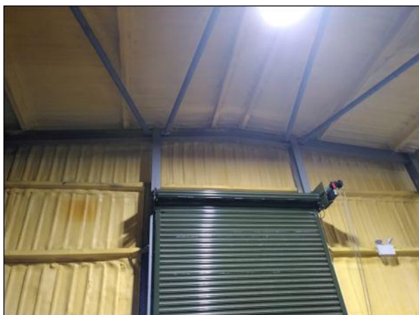
Photo 13: Building 1, internal area, northern end
