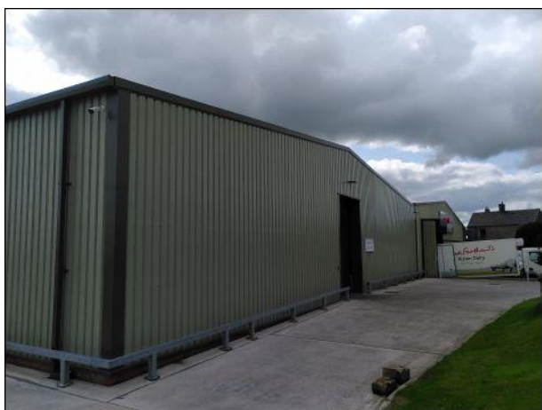
Photo 11: Building 1, western elevation, northern end
