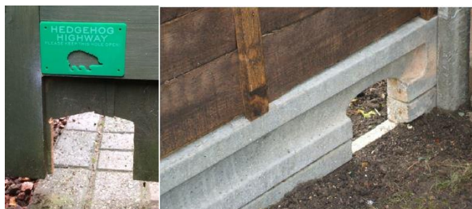
Insert 3: Showing wildlife access gap within fencing
