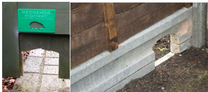
Insert 3: Showing wildlife access gap within fencing
