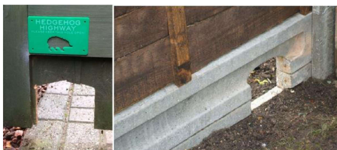
Insert 3: Showing wildlife access gap within fencing
