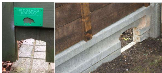
Insert 3: Showing wildlife access gap within fencing
