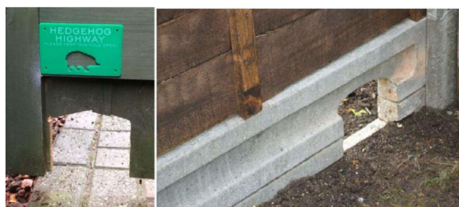
Insert 3: Showing wildlife access gap within fencing
