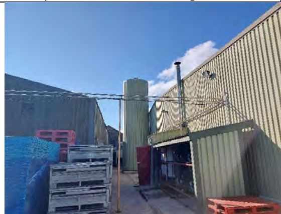
Photo 18: Elevated pipework which transports the milk from the Farm to the left/west to the Dairy to the right/east. Taps at both ends need to be opened for milk flow. Facing south.
