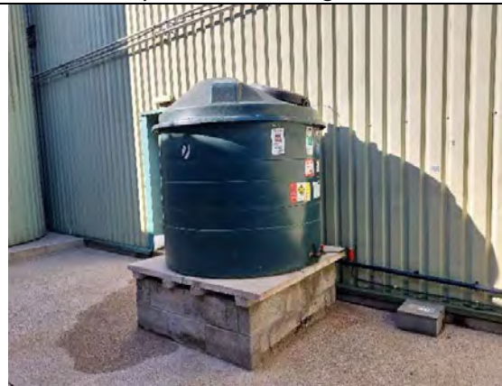
Photo 24: Diesel tank, linked to the boiler for the refrigeration units. No evidence of spills or leaks. Liquid on the surface is water coming from doorway to the left. Facing southwest.
