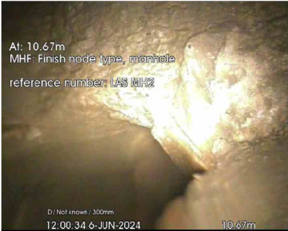
LAS MH1 DOWNSTREAM_10-67m_120034.jpg, 00:00:45, 10.67 m Finish node, manhole, reference: LAS MH2
