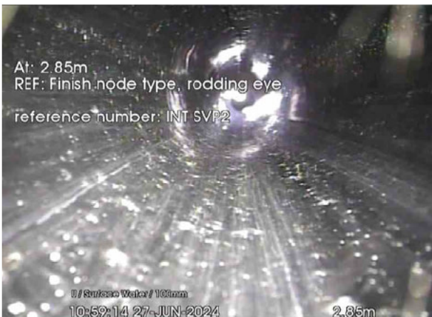
SVP2X_98825d60-1e10-42d7-bb01-43dc20d75285_20240701_111520_547.jpg, 00:00:43, 2.85 m Finish node, rodding eye, reference: SVP2
