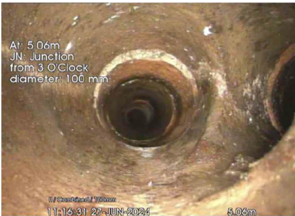
FWMH2 X_22276596-e44d-49d6-a475-e190d659ff31_20240701_1134 17_721.jpg, 00:00:36, 5.00 m
