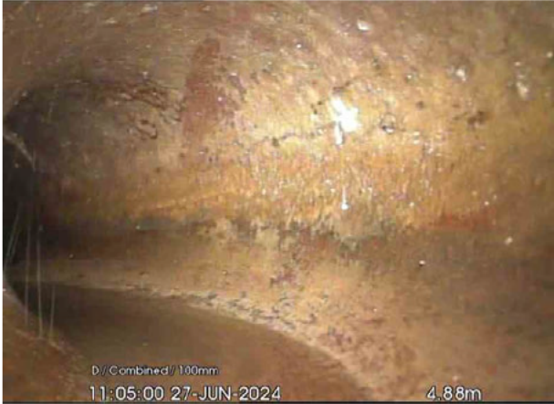
FW1X_d727e8f7-324f-46d0-bd4d-9c4379ebcba6_20240701_112223_537.jpg, 00:01:04, 4.88 m Line deviates left
