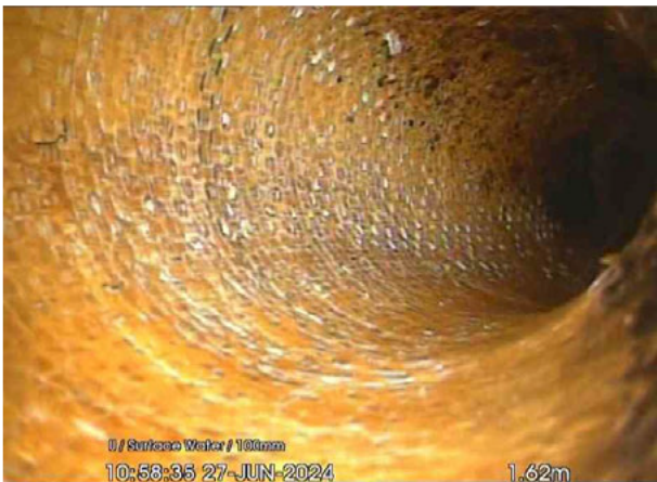
SVP2X_48ccf77e-3fbd-4496-a897-860cc392df7d_20240701_111435_081.jpg, 00:00:27, 1.62 m Line deviates right
