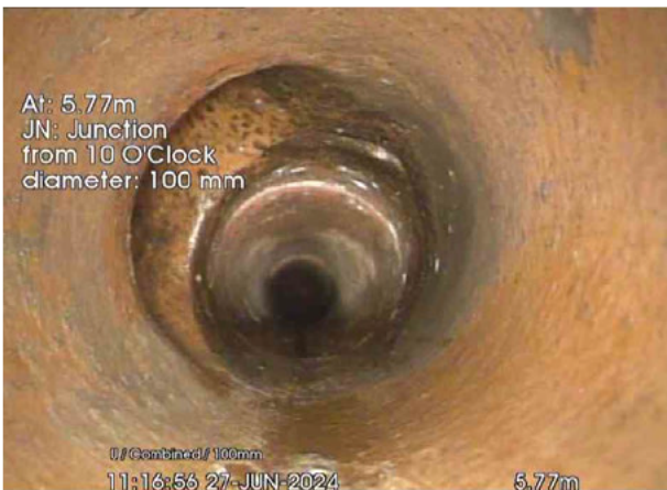
FWMH2 X_b0f54e4a-a9f9-47c2-8a9c-b65a013e21b5_20240701_1135 03_072.jpg, 00:00:44, 5.77 m
