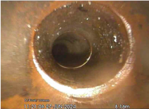
FWMH2X_1f0b3a0f-5a8d-48b4-80d4-6a6671c7ef15_20240701_114204_329.jpg, 00:00:49, 8.16 m Joint displaced, large
