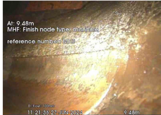
FWMH2X_7d2155c6-75ee-4659-b6dd-f5c55e605b5a_20240701_114239_192.jpg, 00:01:03, 9.48 m Finish node, manhole, reference: FWMH3
