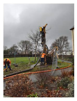
Once the borehole has been drilled the flow and return pipes are installed along its entire length (as shown in the following photograph) and then the gap between the pipe and the borehole is grouted (as required). Once the work is completed and the borehole pipes are connected by underground trench to the property there remains no visible presence on the surface once the works have been completed and the surface treatment has been re-instated, or the grass / vegetation has grown back.
