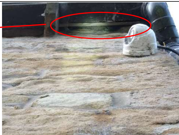
Photo 7: Gap beneath fascia board
