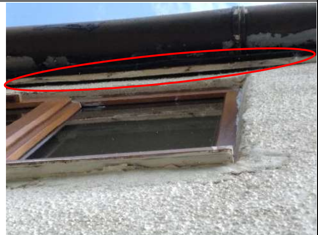
Photo 3: Gap beneath fascia boards on southern elevation
