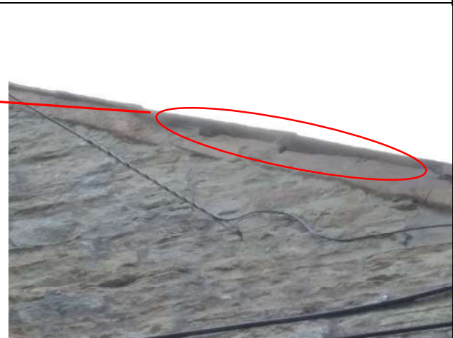
Photo 3: Gap beneath fascia boards on southern elevation
