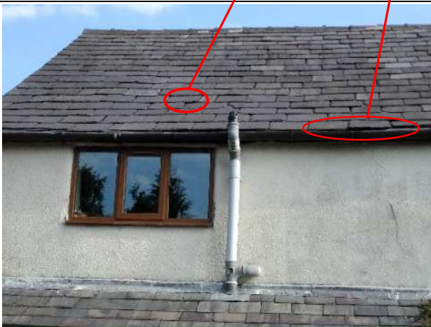
Photo 2: Lifted slates & gaps beneath slates
