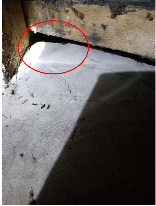
Photo 15: Gap at the top of the dividing wall above the bat droppings
