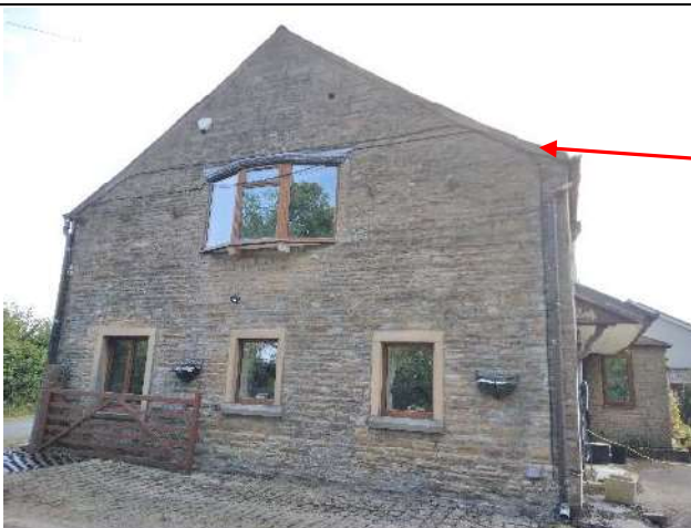
Photo 2: Lifted slates & gaps beneath slates
