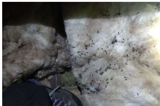
P9: Accumulation of droppings under central tie beam in northern loft area.
