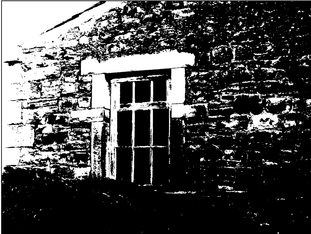
Plate 25: Timber framed 9 light casement
