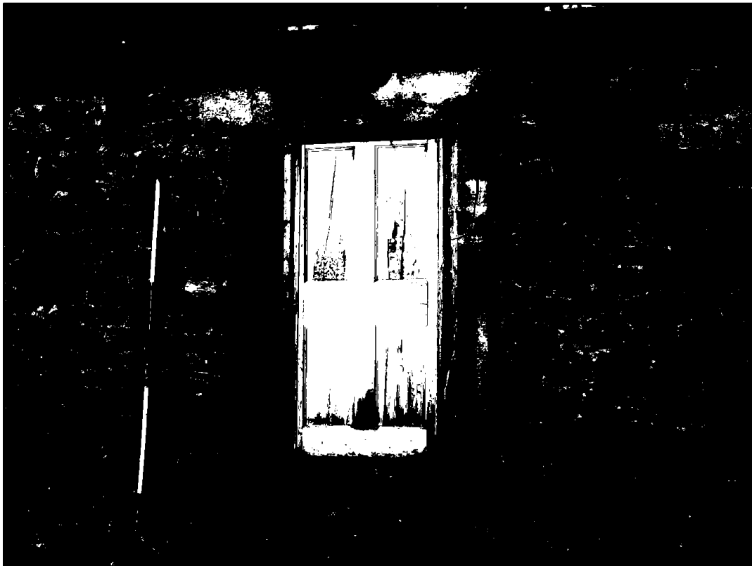
Plate 8: Window with reused timber door as shutter
