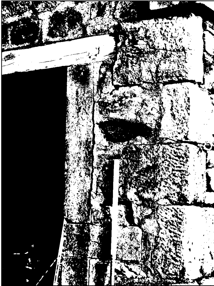
Plate 11: Detail of door jamb and quoins shown above
