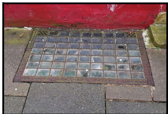
Pavement light on York Street
