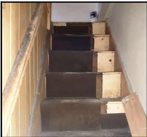
Staircase at first floor level
