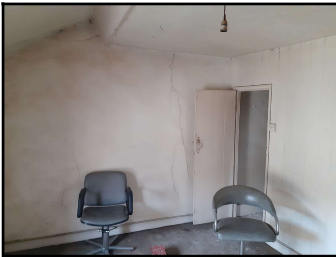
Party wall at second floor level
