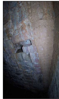
EXTERNAL BRICK TO INTERNAL STONEWORK TIE IN
