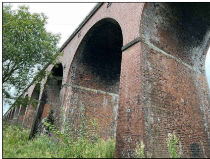
PHOTO 03 VIEW ON PIER 36
