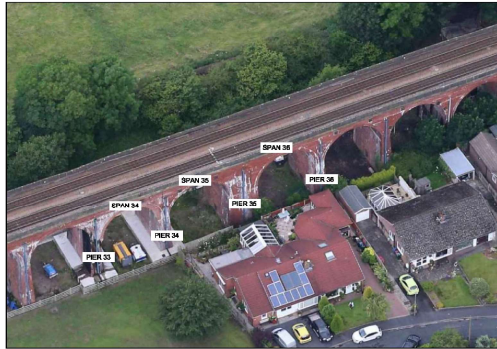
PHOTO 02 PARTIAL AERIAL VIEW ON VIADUCT
