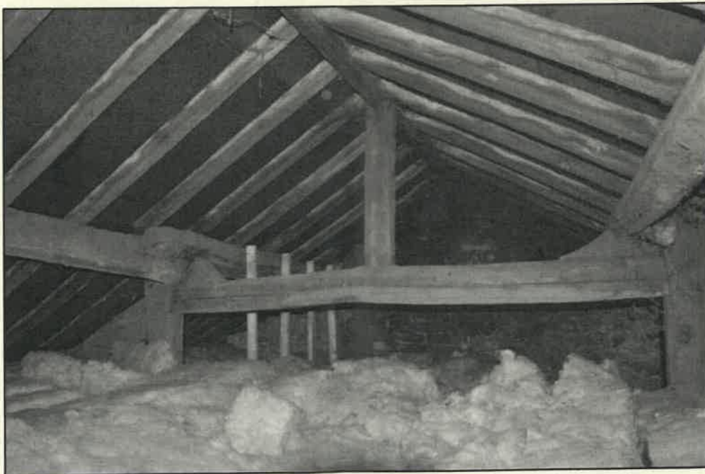
Image of showing roof void showing timber roof supports and bitumastic hessian roof liner. The roof void at 23 Smith Row provides suitable conditions (draught free, dark, undisturbed space) for use by roosting bats.
