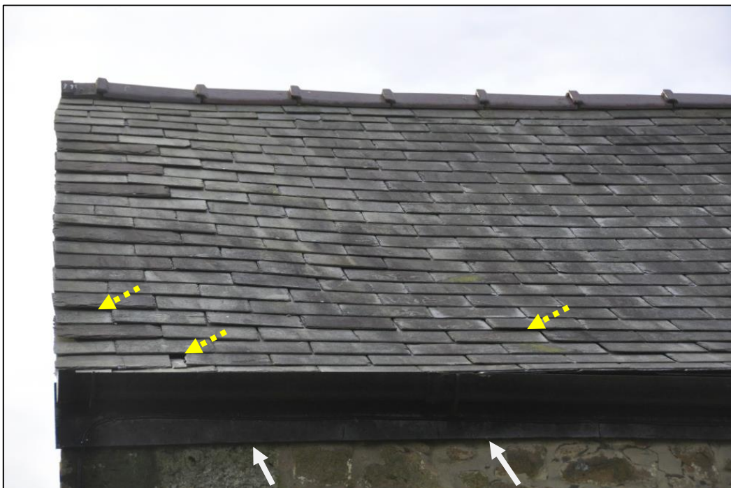
Image of rear roof and roof edge. Note gaps between slates (yellow dashed arrow) and timber fascia (white arrow). These features provide high potential bat roosting and bat access points on this building.
