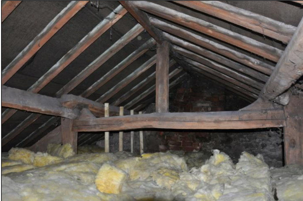
Image of roof void showing timber roof supports and bitumastic hessian roof liner. The roof void at 23 Smithy Row provides suitable conditions (draught free, dark, undisturbed space) for use by roosting bats.
