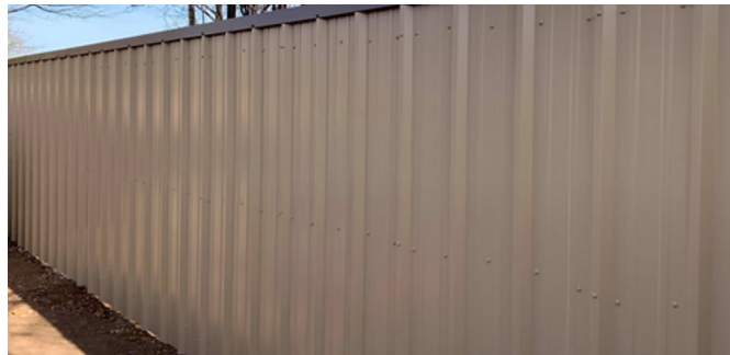
Corrugated metal fencing
