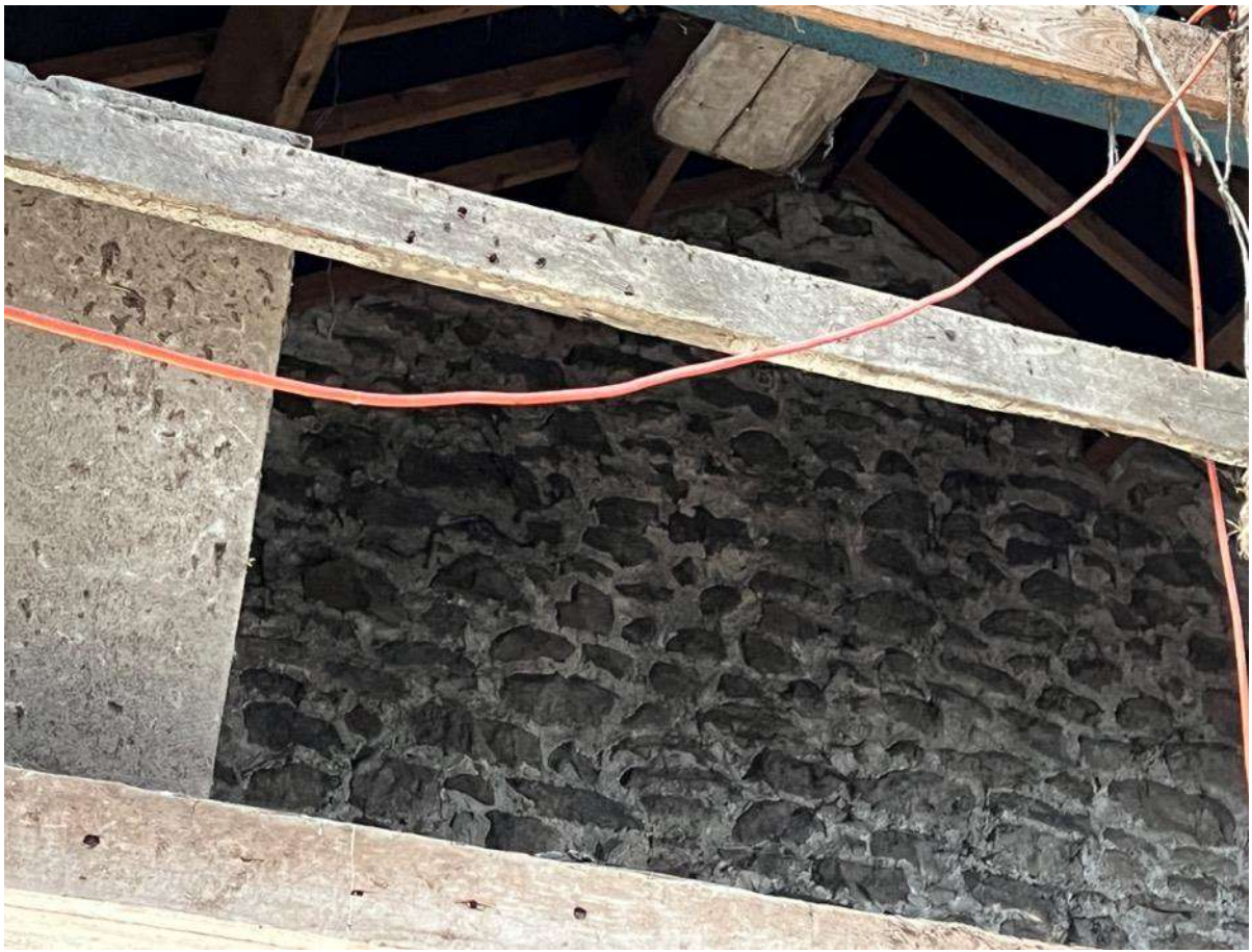
Photo 41 – Internal looking west to gable with house
