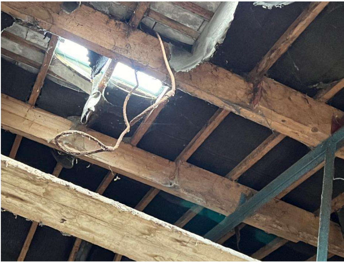
Photo 39 - Internal roof truss and timber purlins & rafters
