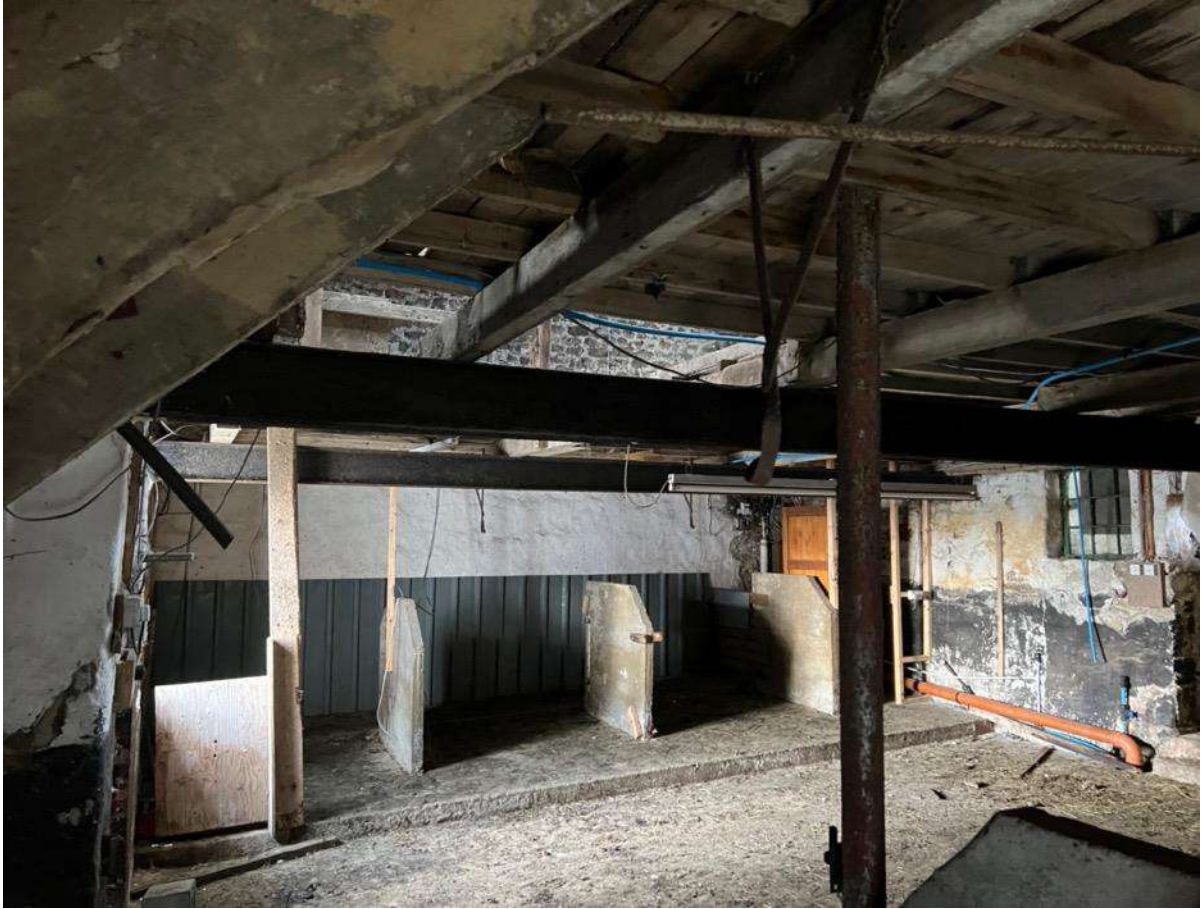
Photo 22 – Internal looking to gable with house (west)
