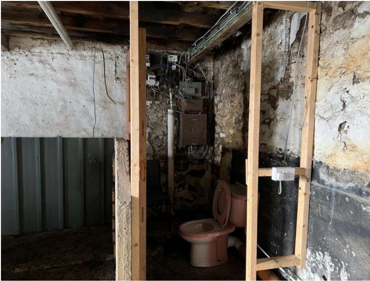
Photo 32 – Internal north west corner with toilet
