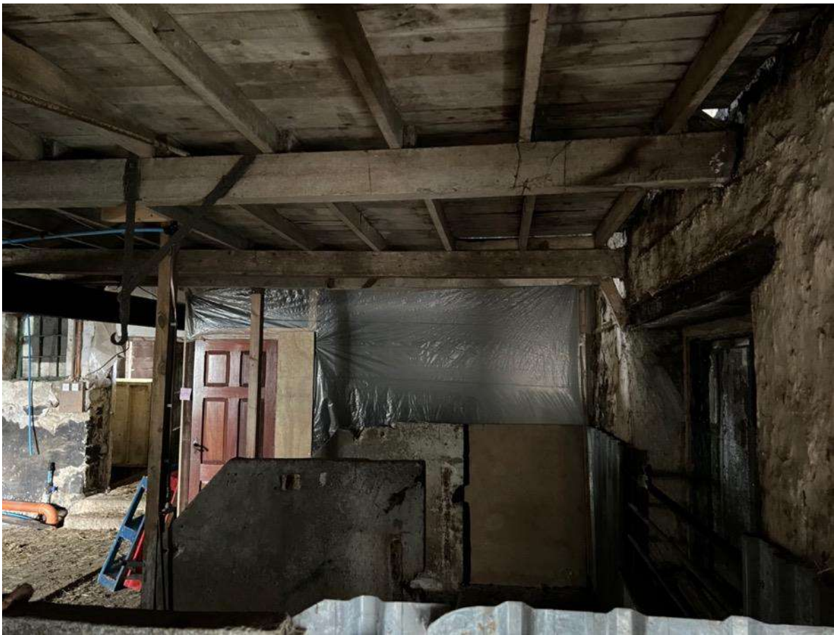
Photo 23 – Internal looking north
