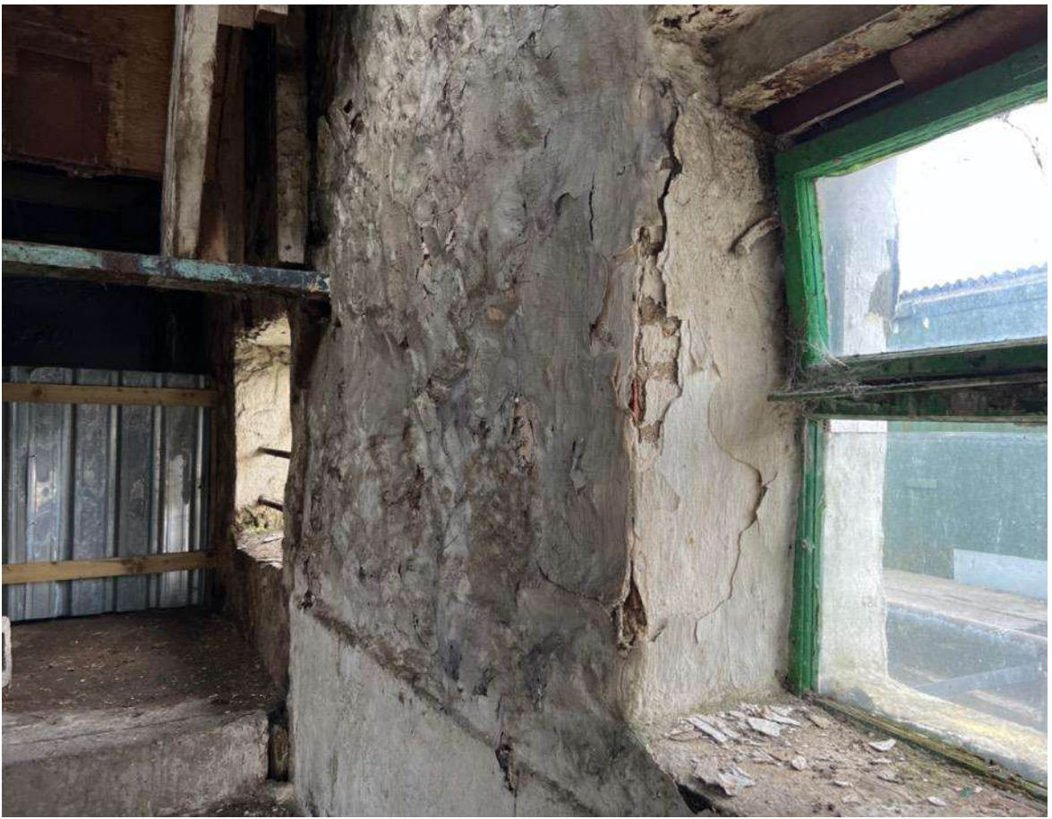
Photo 19 - Internal south outrigger
