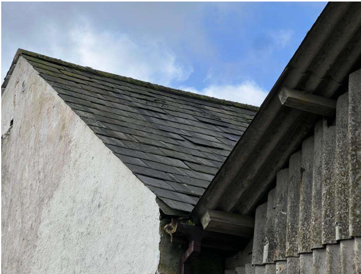
Photo 15 - North Elevation roof
