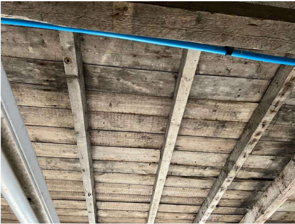
Photo 35 – Internal loft timbers
