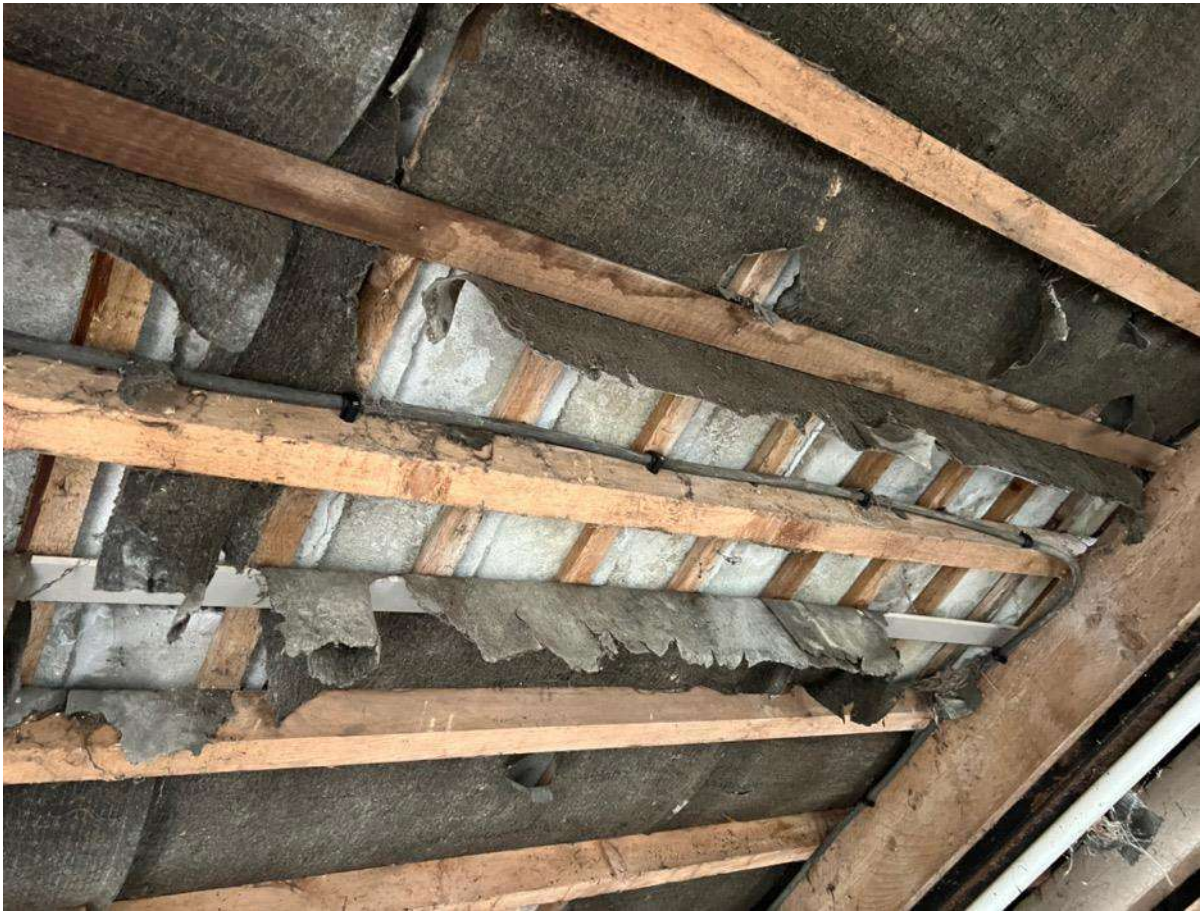
Photo 18 - Internal south outrigger
