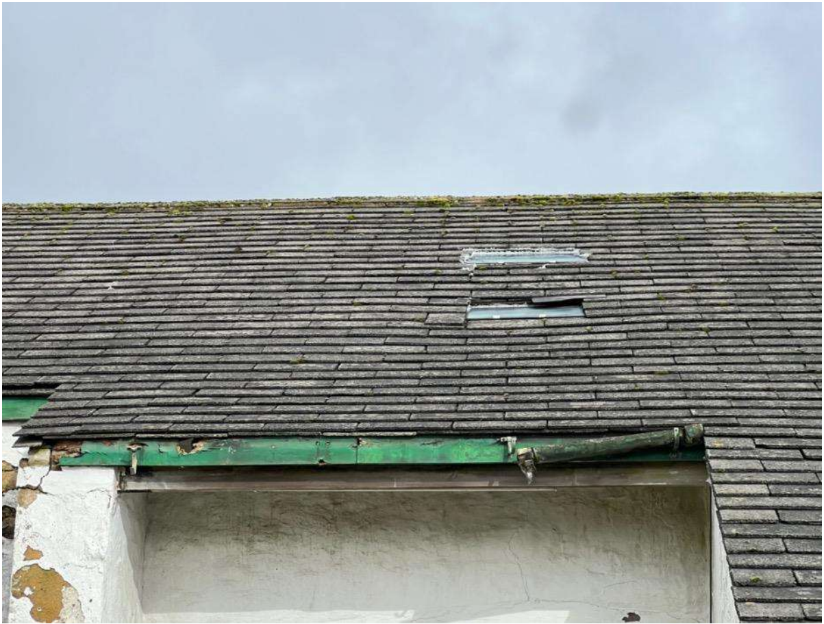
Photo 4 – South Elevation roof
