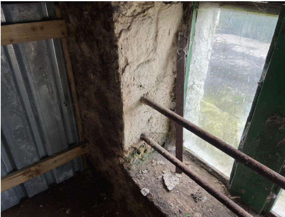
Photo 25 – Internal east gable
