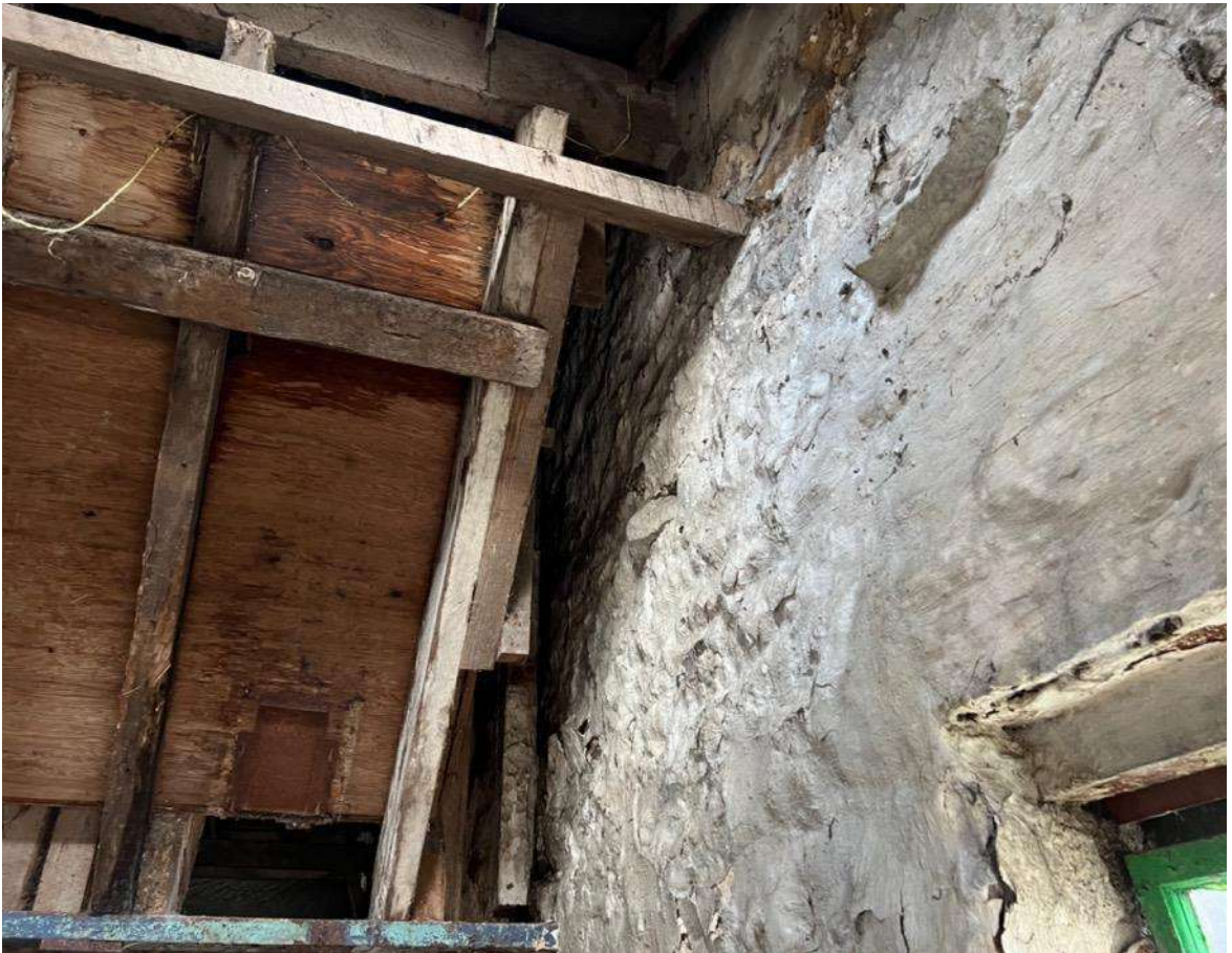
Photo 20 - Internal south outrigger
