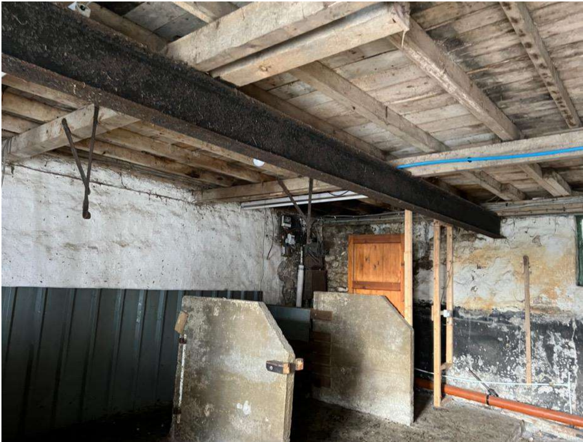
Photo 26 - Internal looking to gable with house and north elevation
