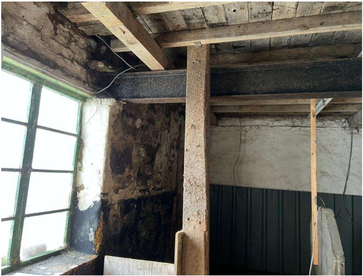
Photo 27 – Internal looking to gable with house and south elevation
