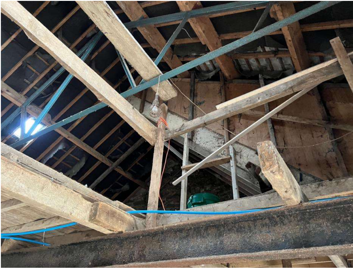
Photo 36 – Internal roof truss
