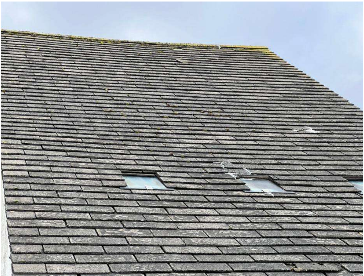
Photo 3- South Elevation roof
