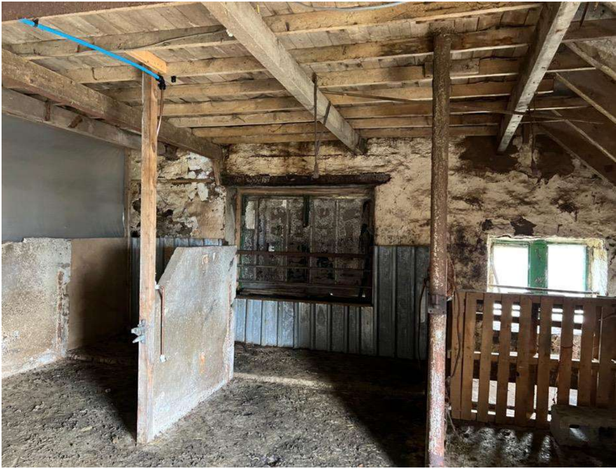
Photo 30 – Internal stalls and loft floor
