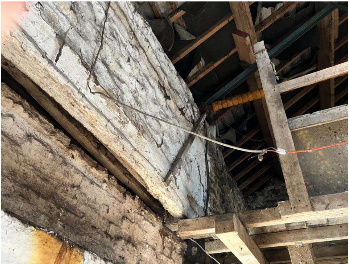
Photo 42 – Internal south elevation
