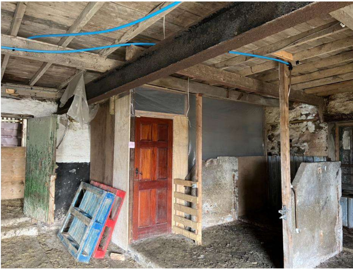
Photo 31 – Internal stalls and loft floor
