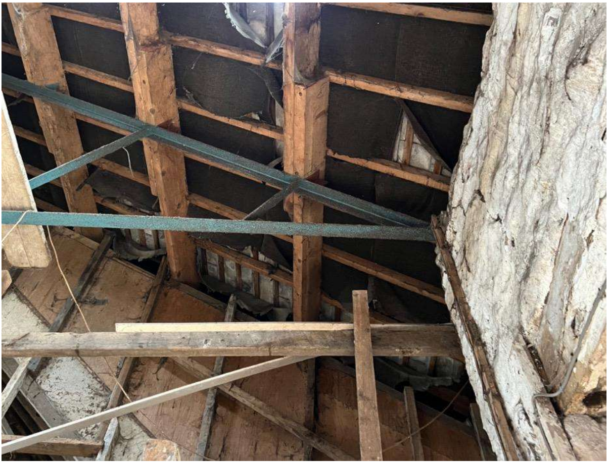
Photo 37 - Internal roof truss and timber purlins & rafters
