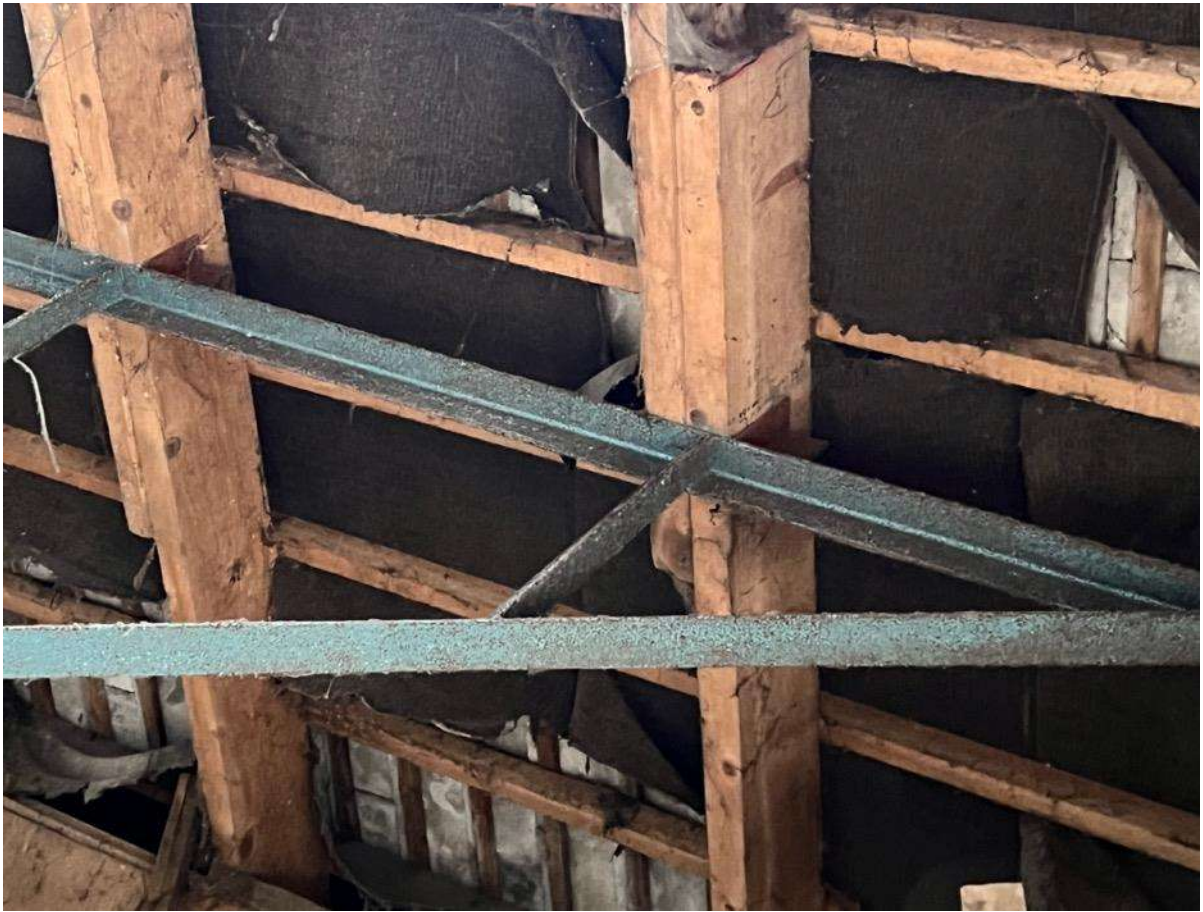
Photo 38 - Internal roof truss and timber purlins & rafters
