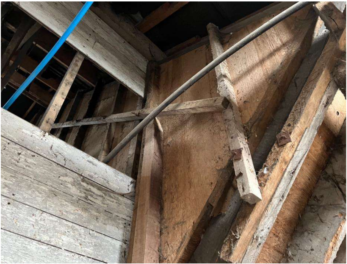
Photo 21 – Internal south outrigger (hopper)
