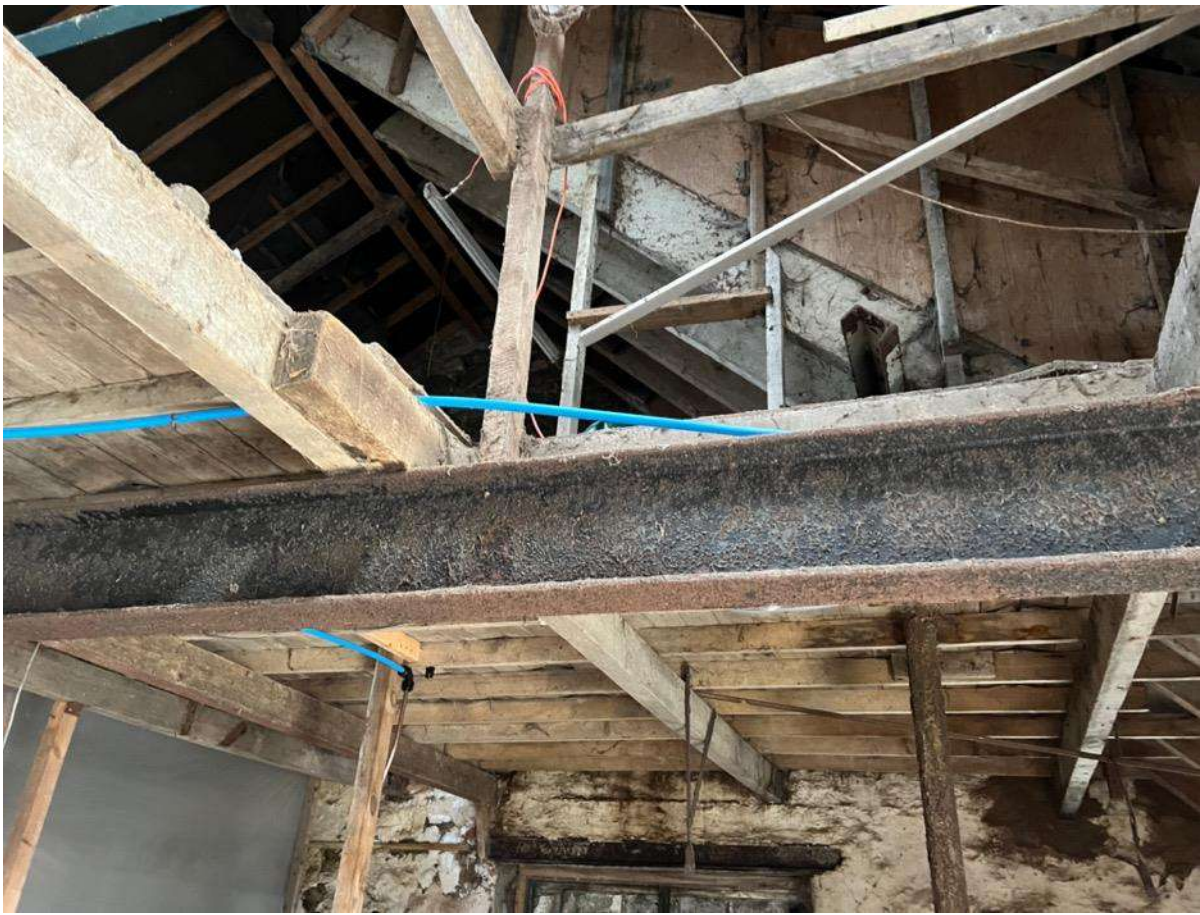
Photo 29 – Internal loft floor and hopper
