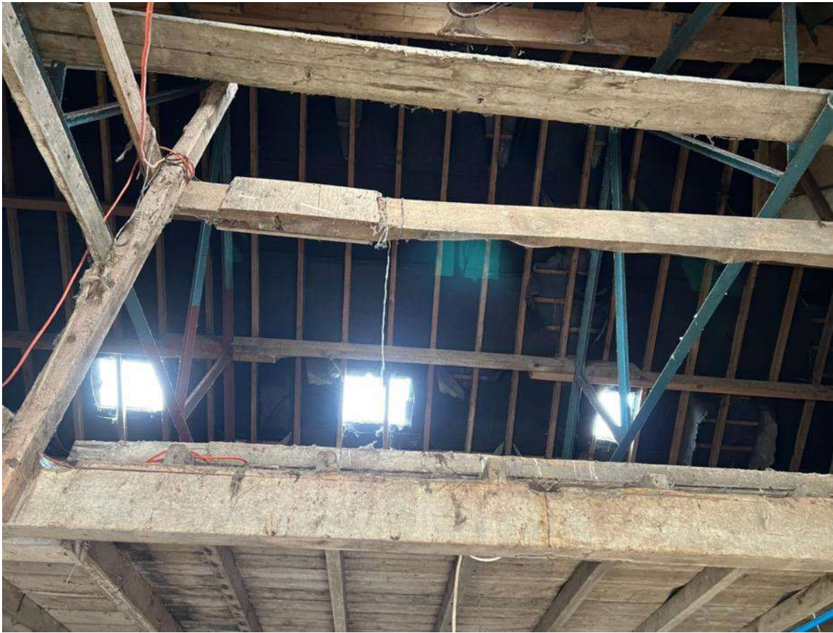
Photo 40 – Internal loft floor and roof structure
