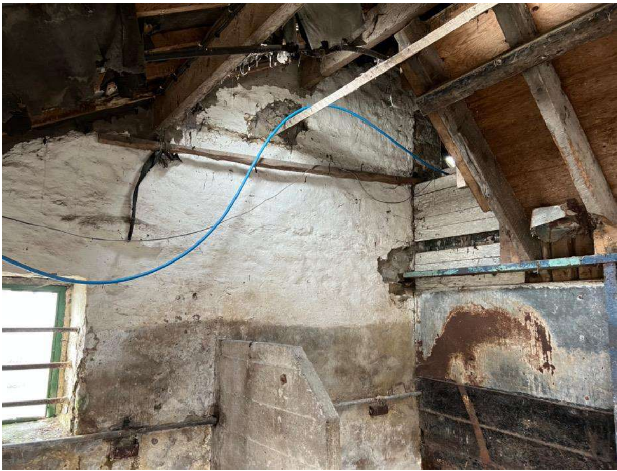
Photo 17 - Internal south outrigger
