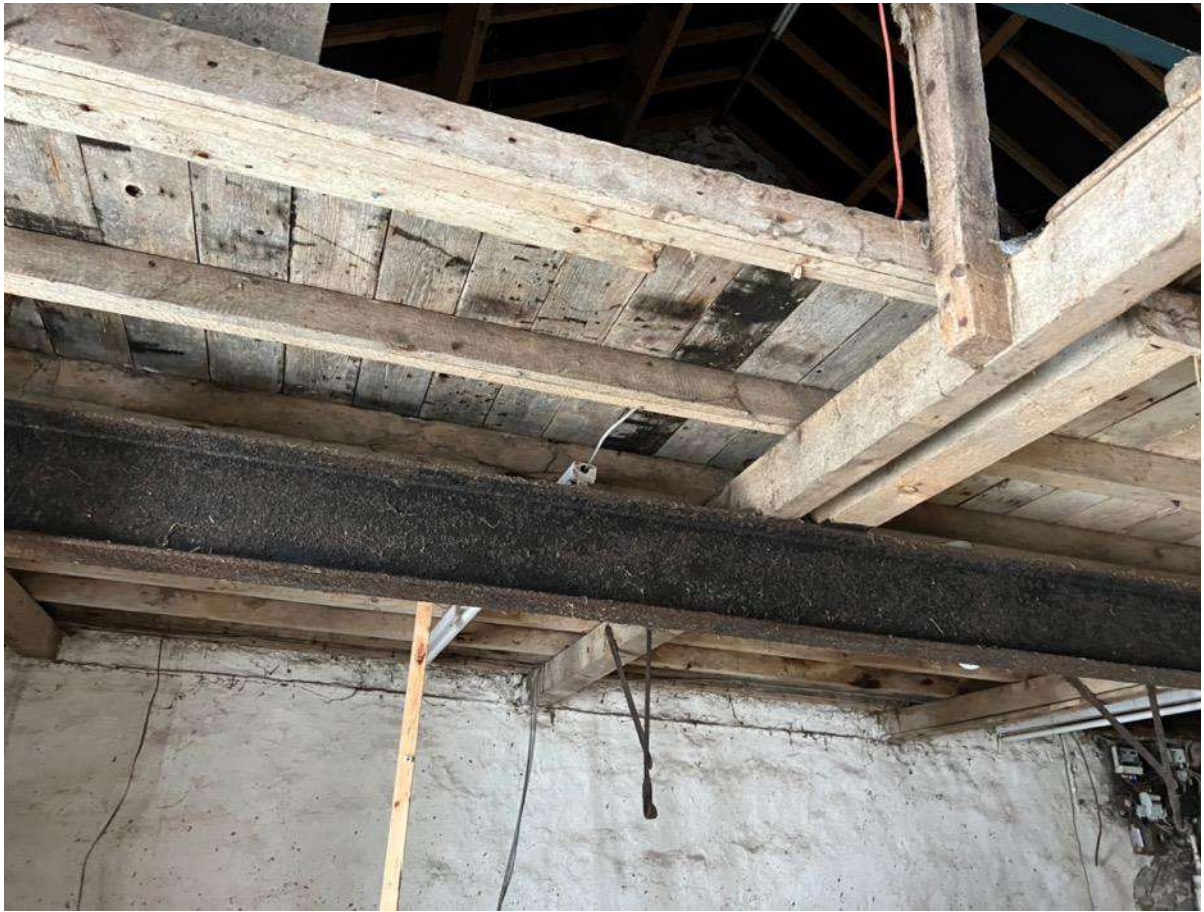
Photo 28 – Internal loft floor
