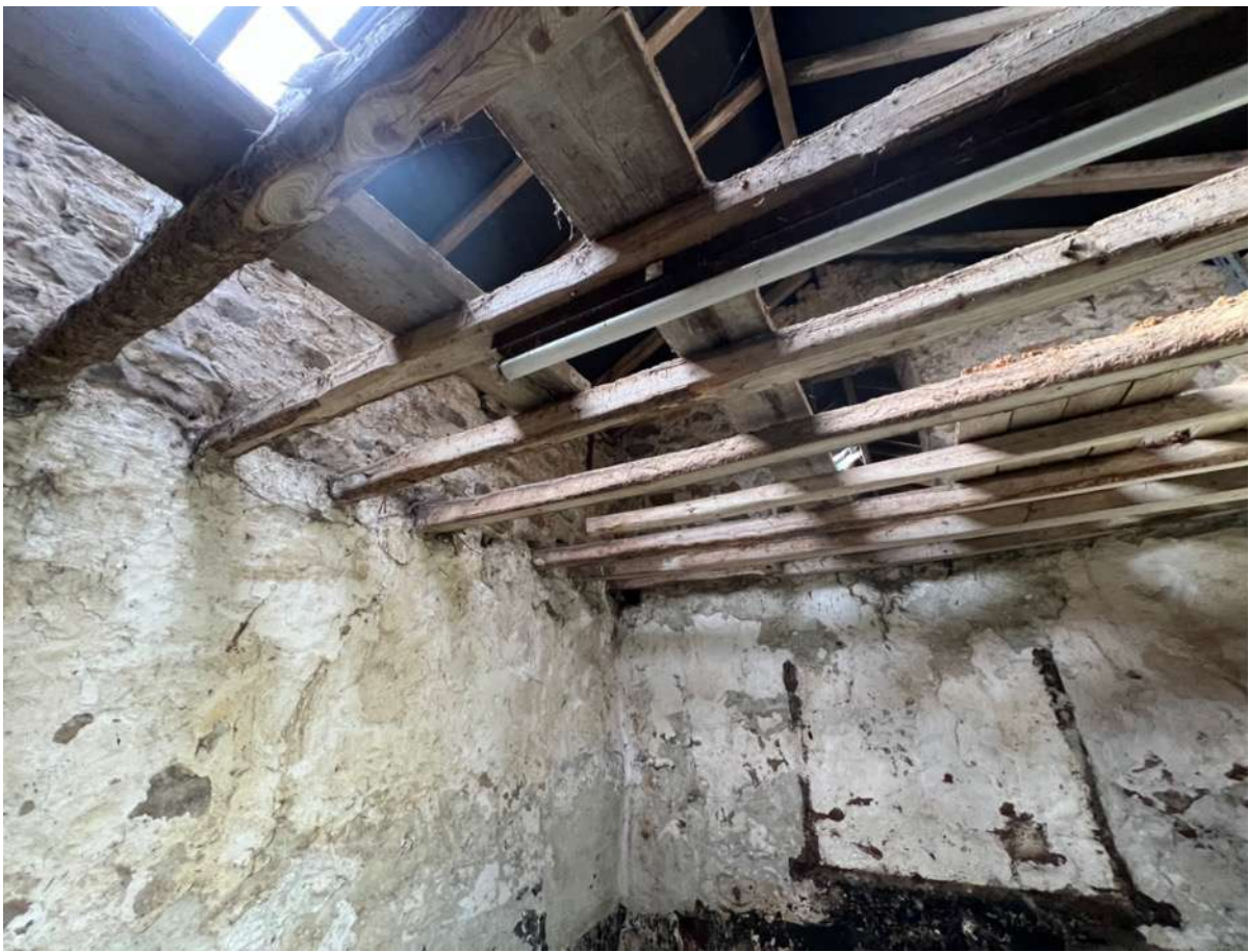
Photo 23 – Internal east end
