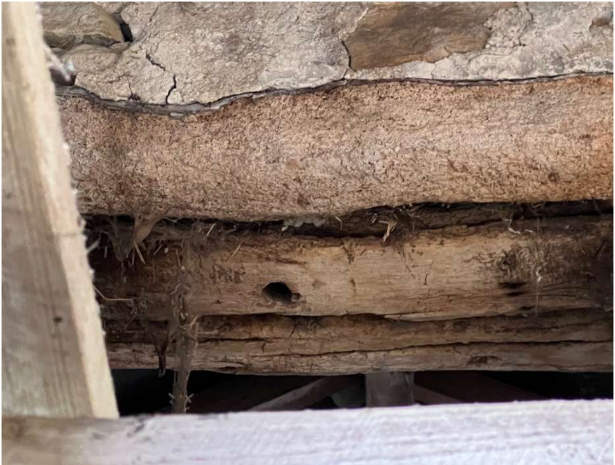
Photo 26 - Timber lintels to mid opening in loft
