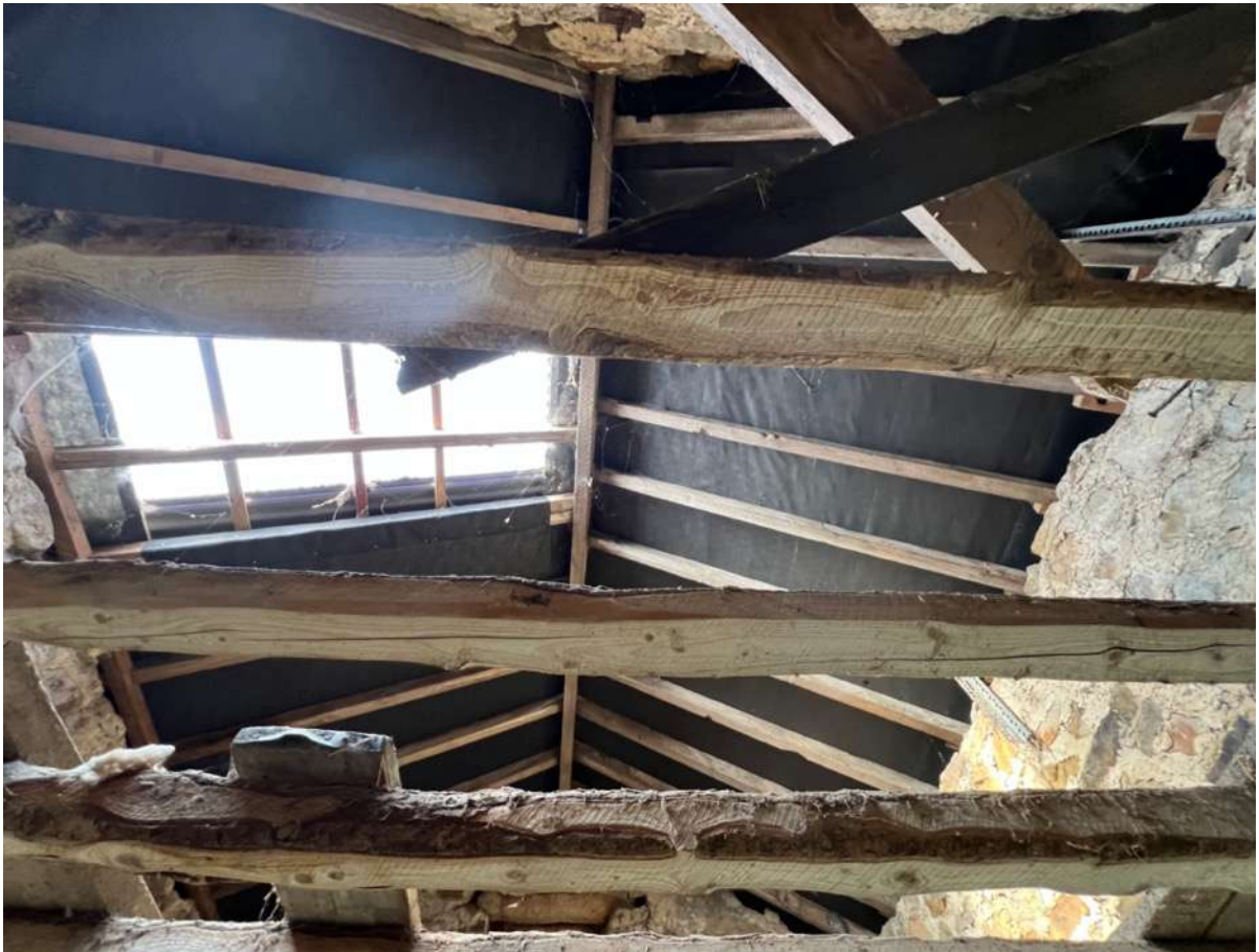
Photo 22 – First floor and roof structure at east end
