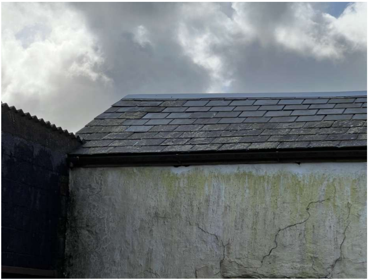
Photo 3- North Elevation and roof
