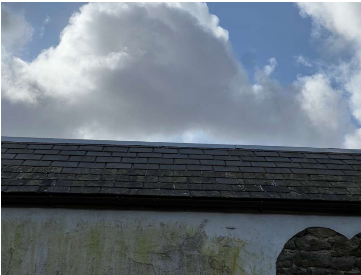
Photo 2 – North elevation roof
