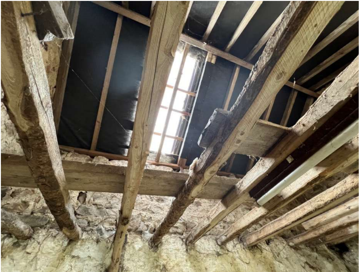
Photo 24 - First floor and roof structure at east end
