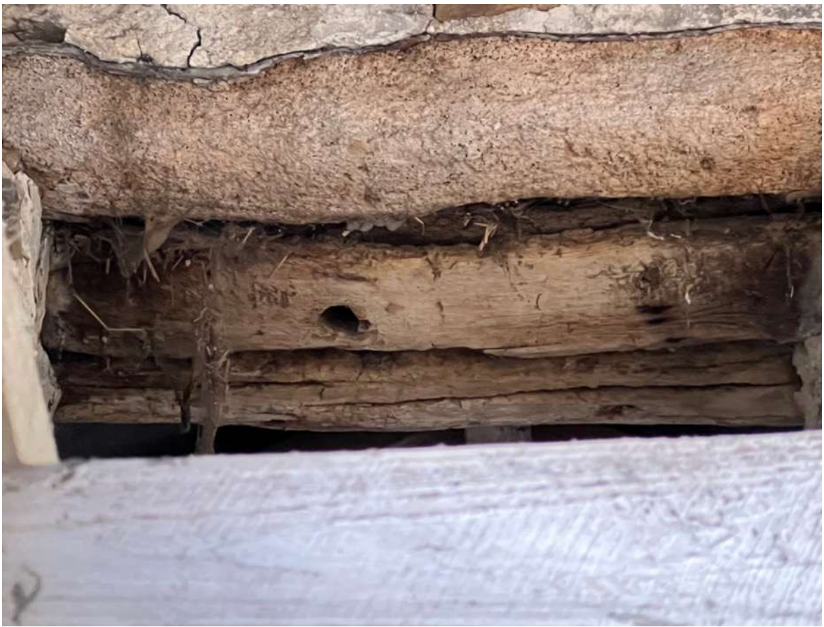
Photo 25 – Timber lintels to mid opening in loft
