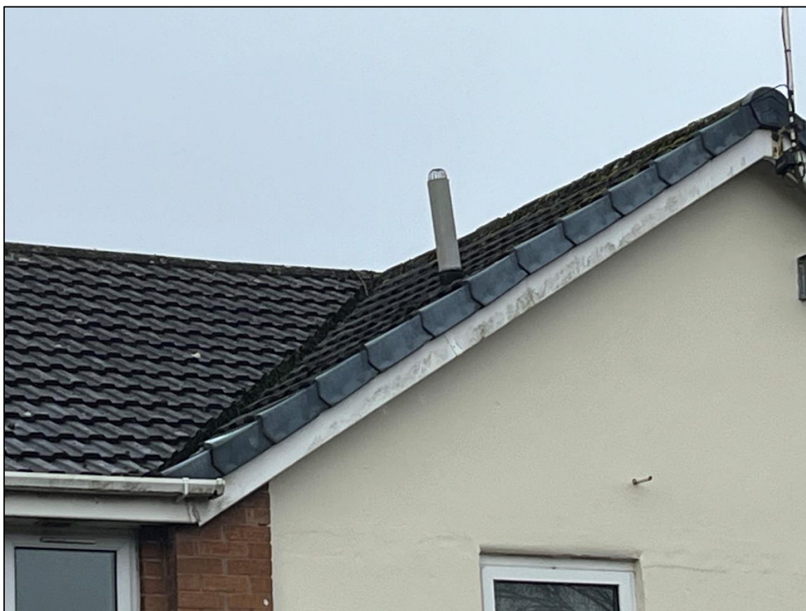
Plate 3 – Tight nature of roof tiles and UPVC capping
