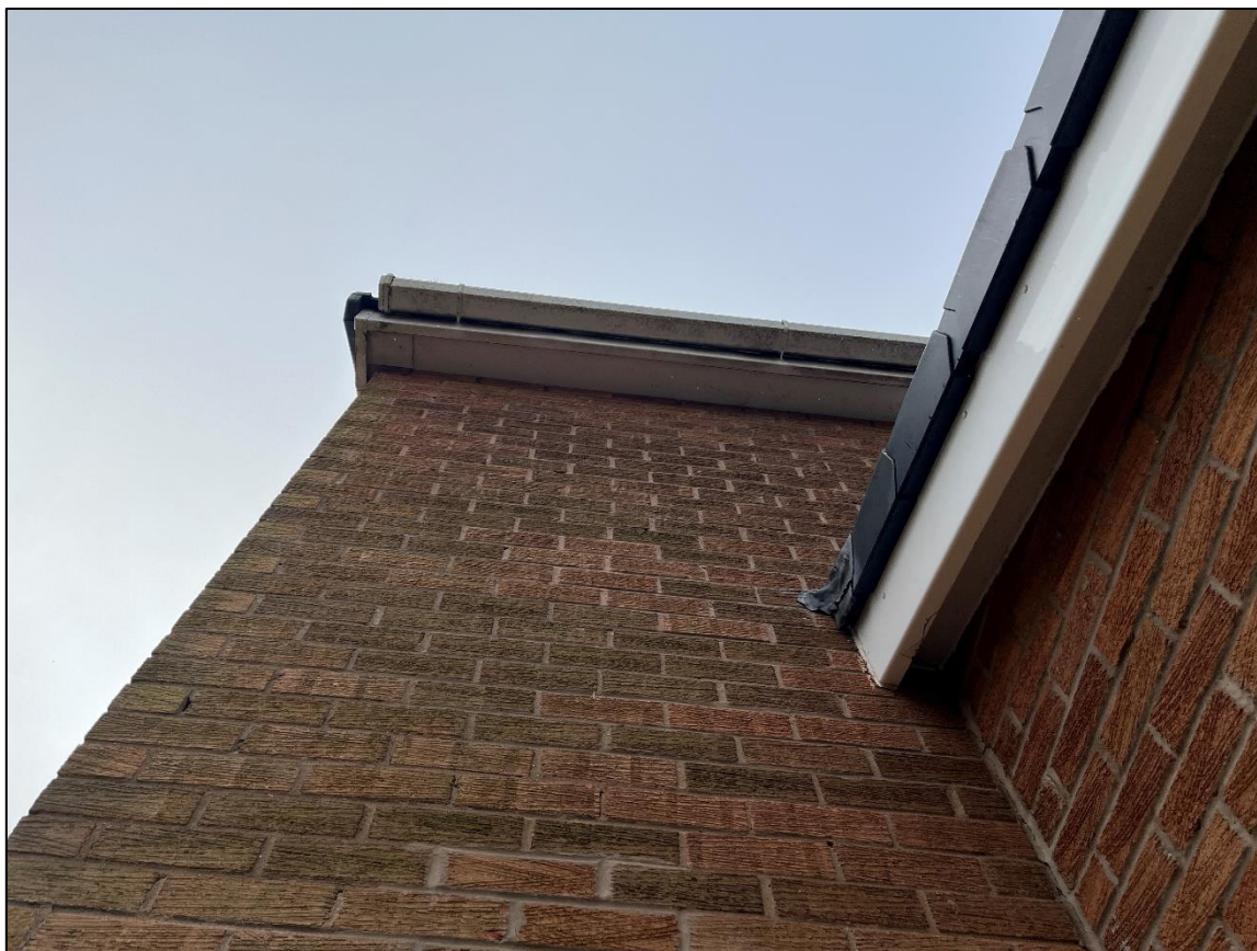
Plate 7 – Tight-fitting nature of soffits
