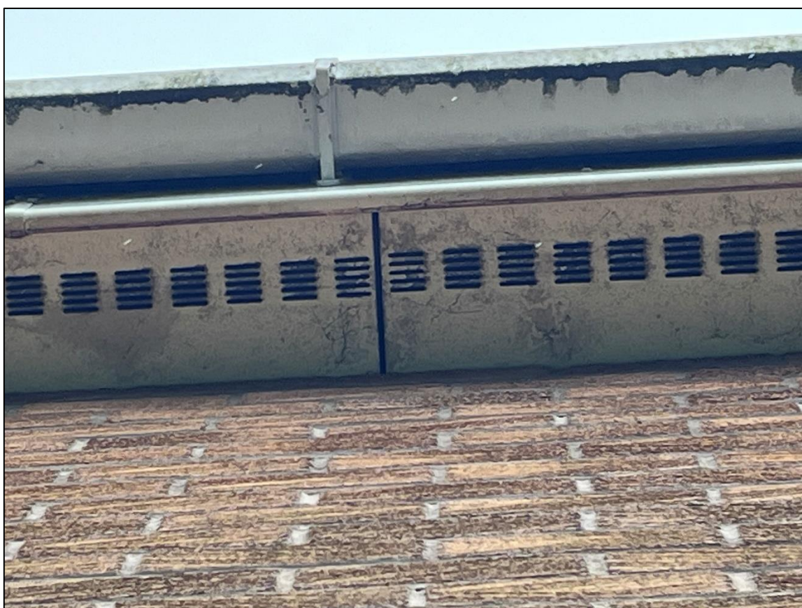
Plate 4 – Nature of the soffit to the south, with potential gap
