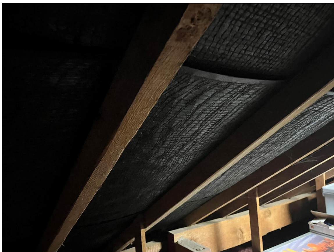
Plate 10 – Bitumen lining within loft space
