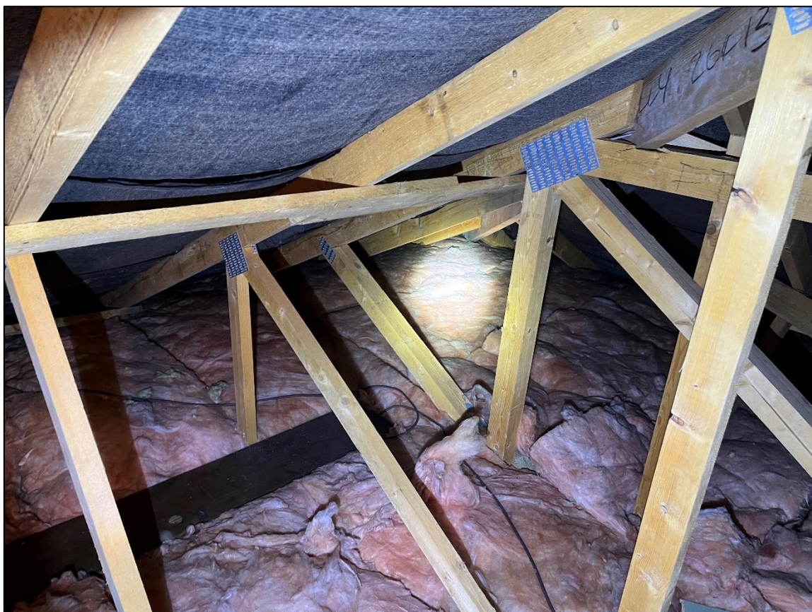
Plate 12 – Character of trussed beam section of loft space
