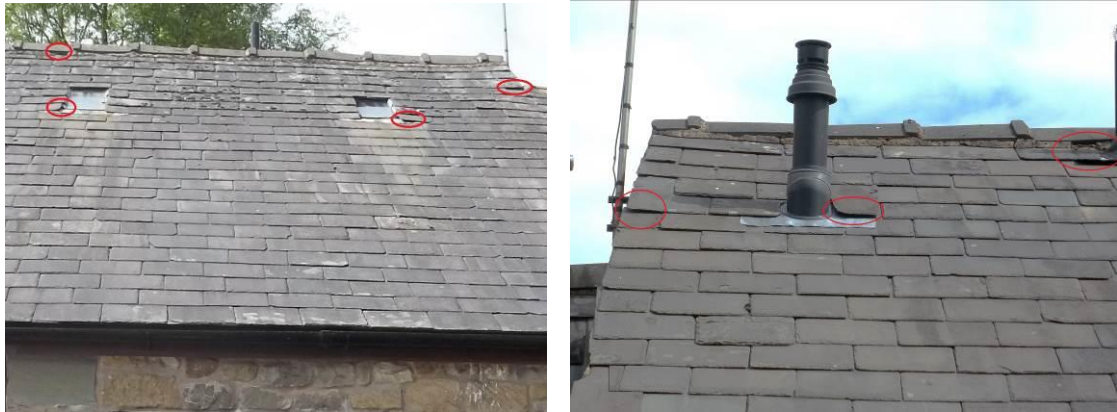
Front and back roof pitches
