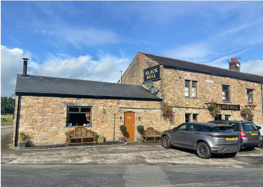
View of the main elevation of the Black Bull
