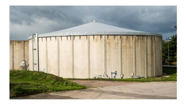
Storage tank covers are made to suit the tank. The materials we are resistant to manure and other aggressive liquids and chemicals. Tensioned over the tank roof with manholes to allow easy access, they are designed these to ensure ultimate protection and coverage. Material is all high frequency welded for integrity load bands every 1000mm from the centre cap to the sides. Heavy-duty straps, ratchet centre pole and hatch covers are all included for a full installation kit.
