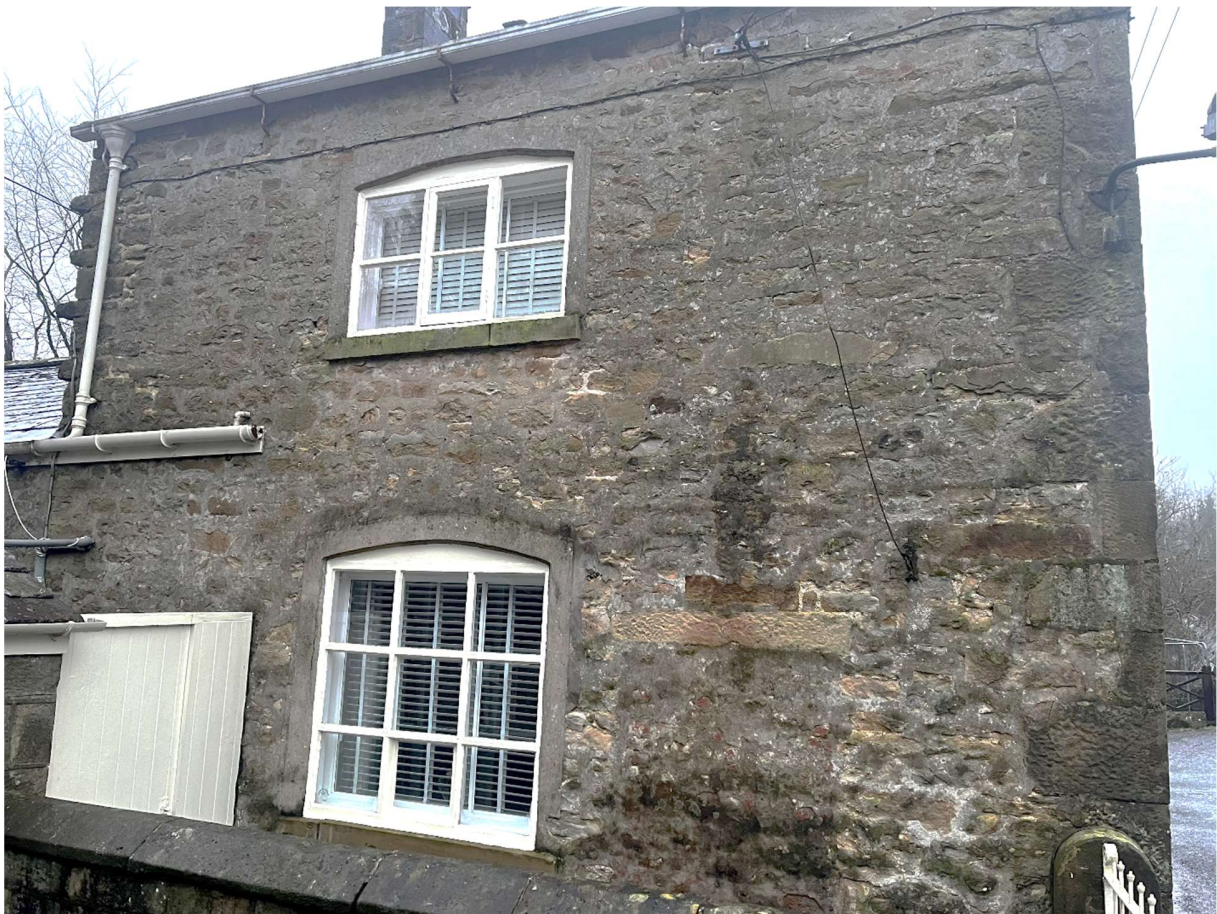
Photo 1 – Rear of the dwelling (north facing)
