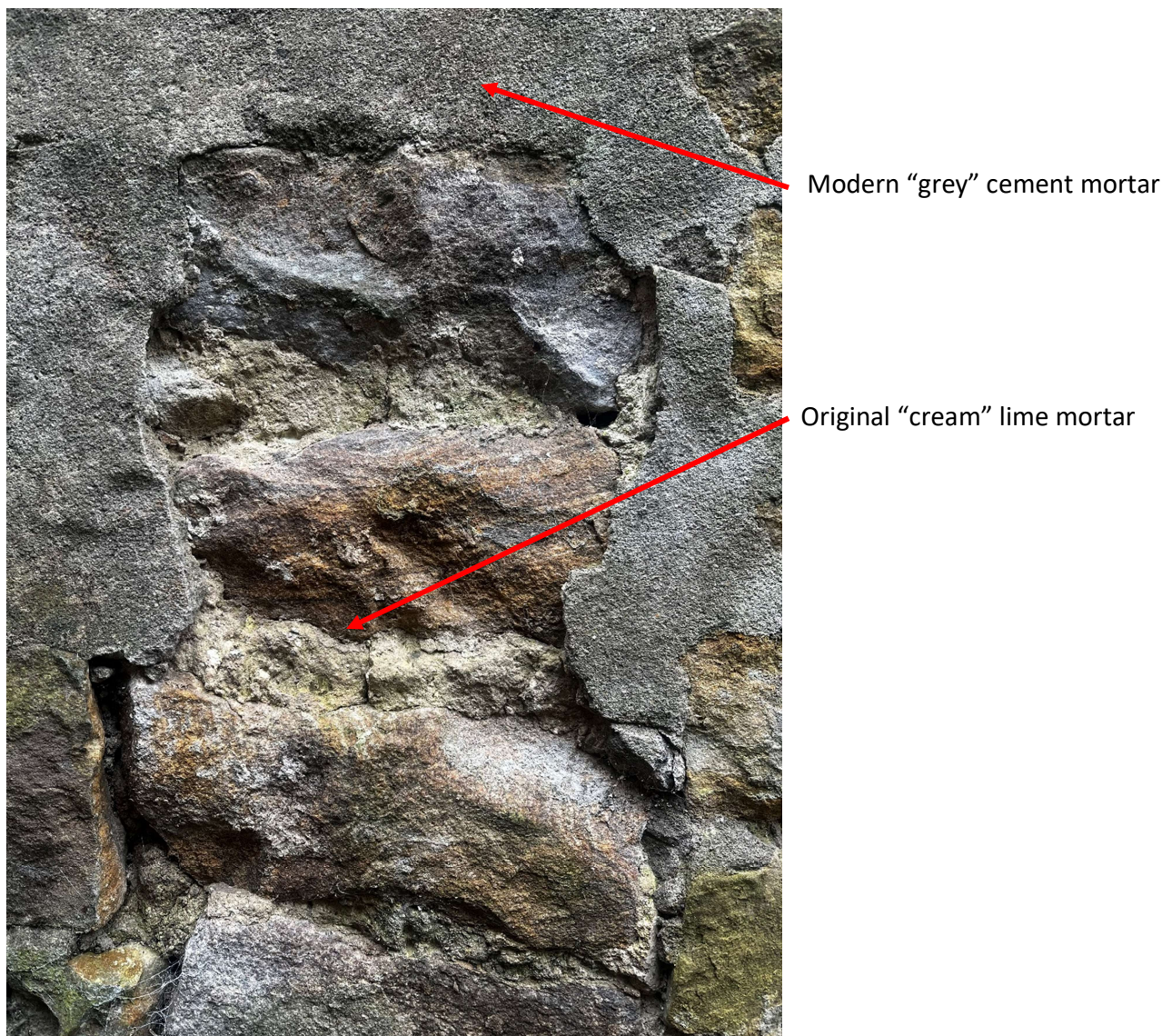
Photo 4 – Original lime mortar evident underneath modern cement mortar
