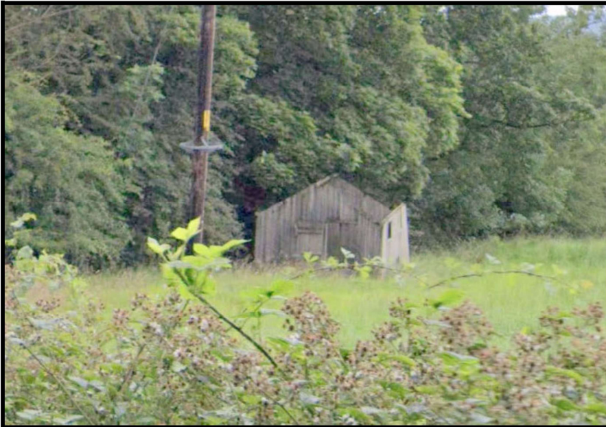
View of shed and electricity supply pole
