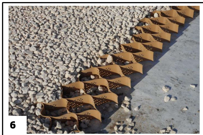
Photo 6: A view of the detail of the GeoWeb™ no dig cellular confinement system. Note the cells, roadstone fill and geotextile base layer.
