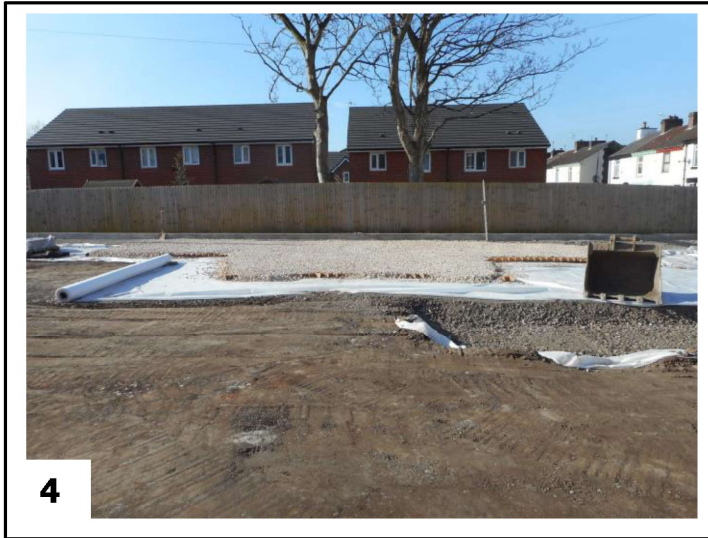
Photo 4: A view of a GeoWeb™ installation for a car parking area to protect the RPAs of two trees.
