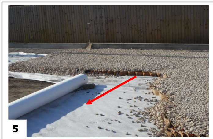
Photo 5: A closer view of the GeoWeb™ surface showing the cells filled with road stone and the geotextile membrane base layer, red arrow.
