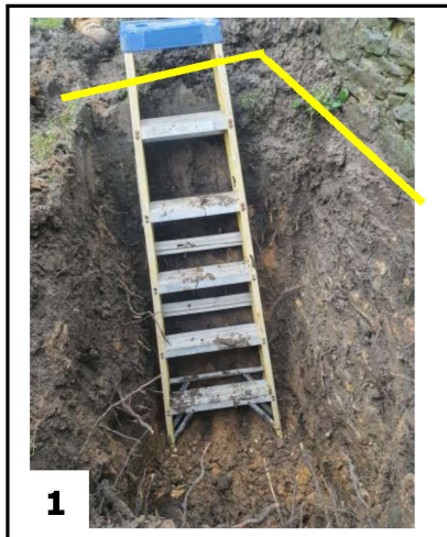
Photo 1: A view of one of the excavated trial pits showing the below ground area of the wall. Ground level is shown by the yellow lines.
