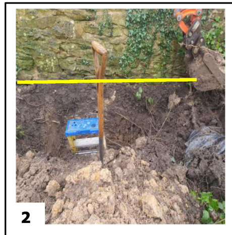
Photo 2: Another view of a trial pit with ground level shown by the yellow line. The small roots in this trial pit are shrub roots. Note no roots are coming through the wall.
