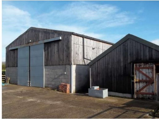
Front of both buildings
