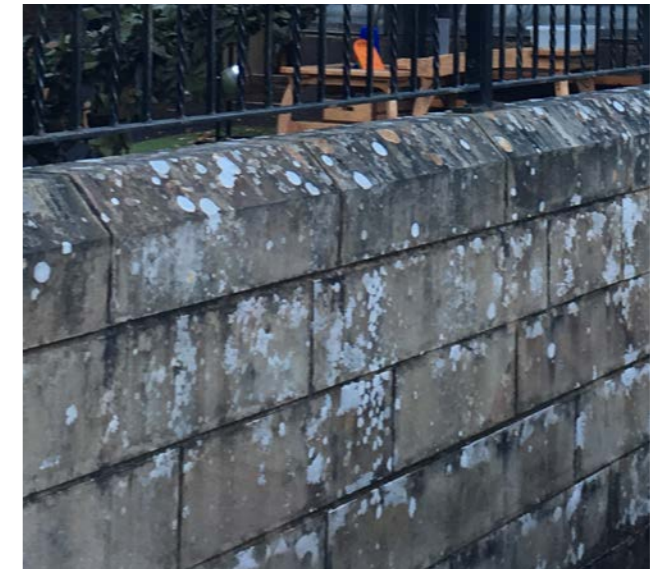
Re-used stone to base of building
