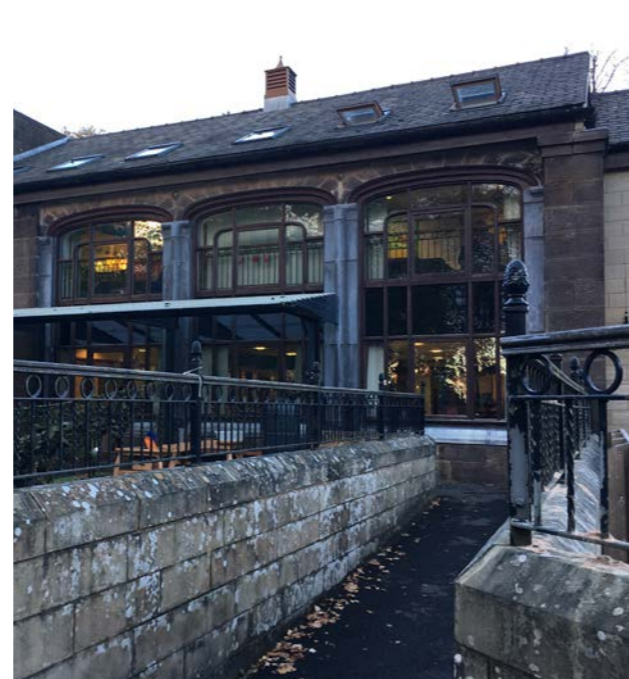
View of existing ramp from the South
