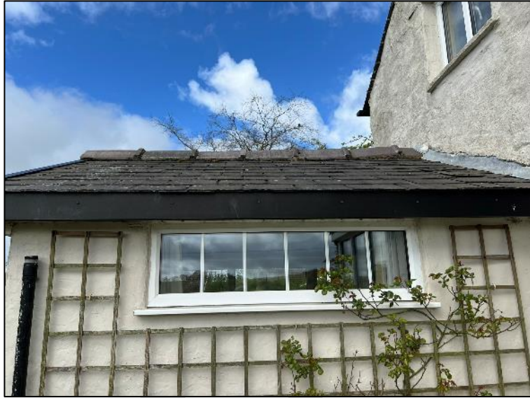
Photo 3: east elevation of the "summer house" extension, showing roof tiles and ridge in good order.
