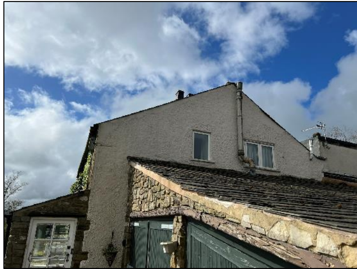
Photo 5: Main dwelling showing traditional stone slates and timber facias with potential for bat roosting.
