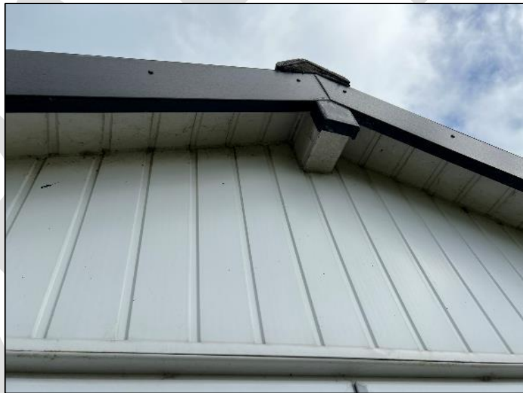
Photo 4: South elevation showing close-up of uPVC cladding and roofline, all in a good state of repair.
