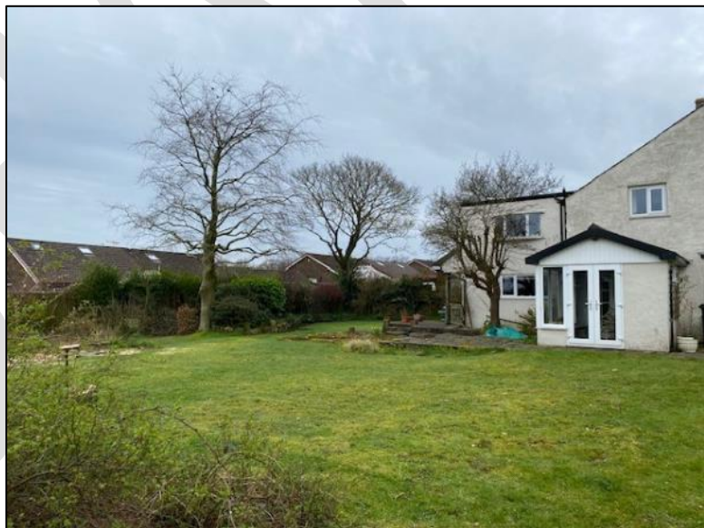
Photo 2: South elevations of the house, showing the single storey extension to be demolished.
