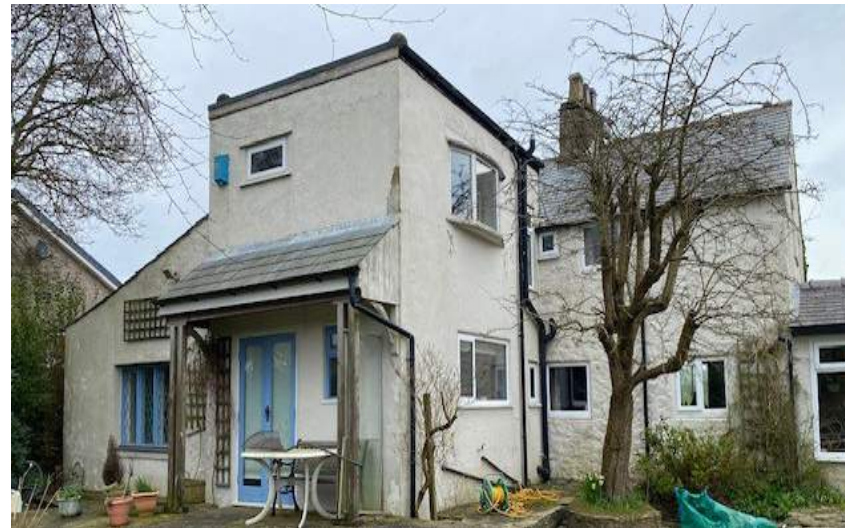
Photo of rear elevation to Moorcot
