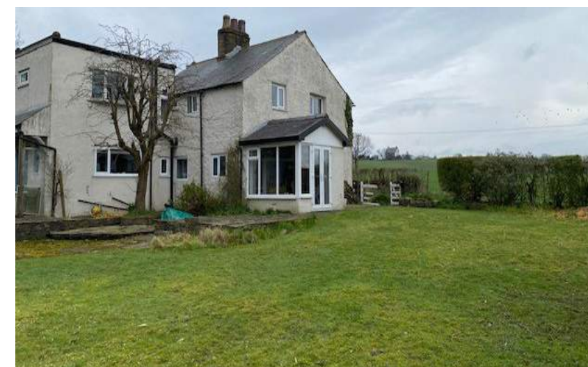
Photo of side elevation to Moorcot
