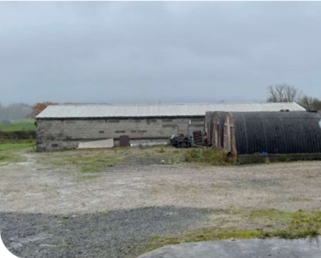
Figure 1.2: Existing north elevation
