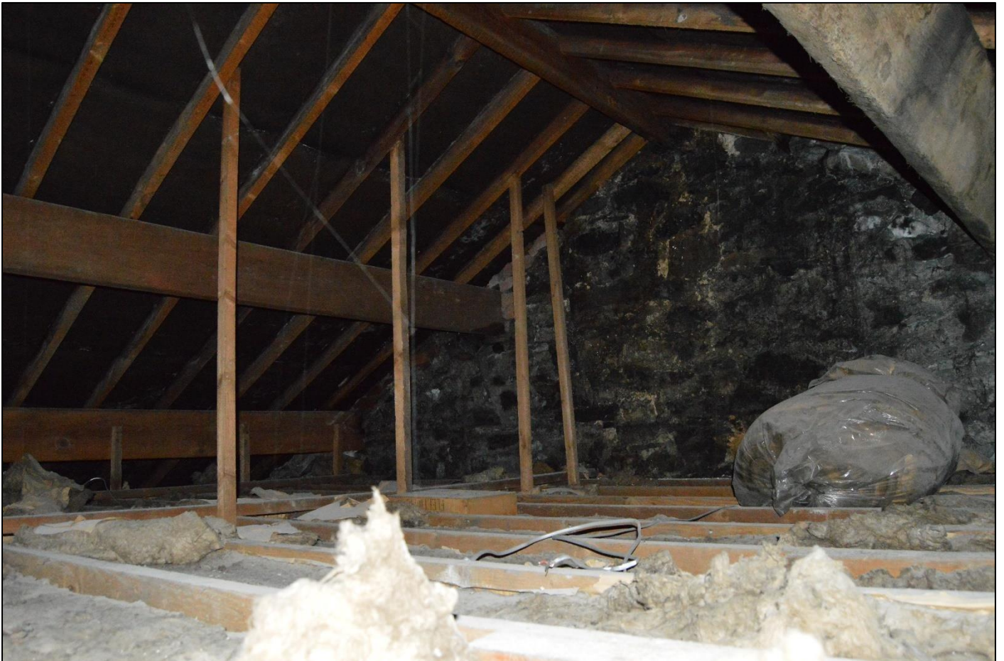
PL24: View of roof structure to the northwest dual pitch roof.
