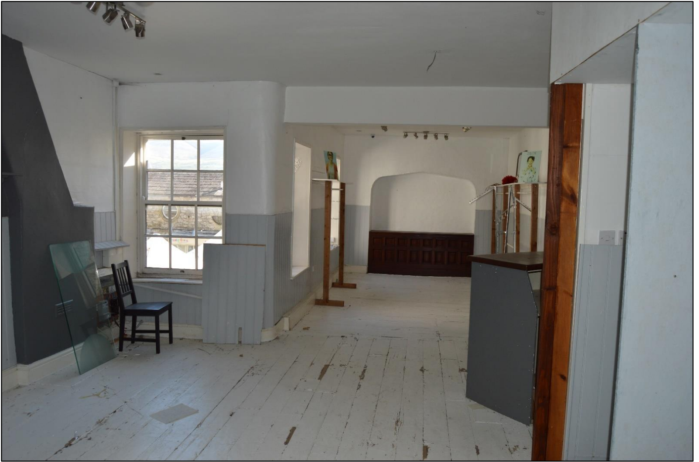
PL19: View southeast within the first-floor shop unit.
