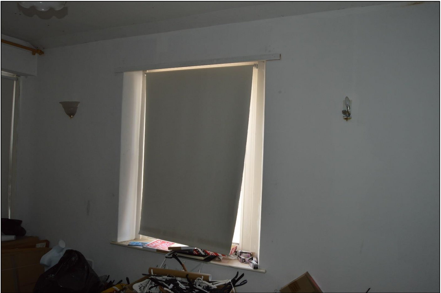
PL22: View northwest within the first-floor front unit.
