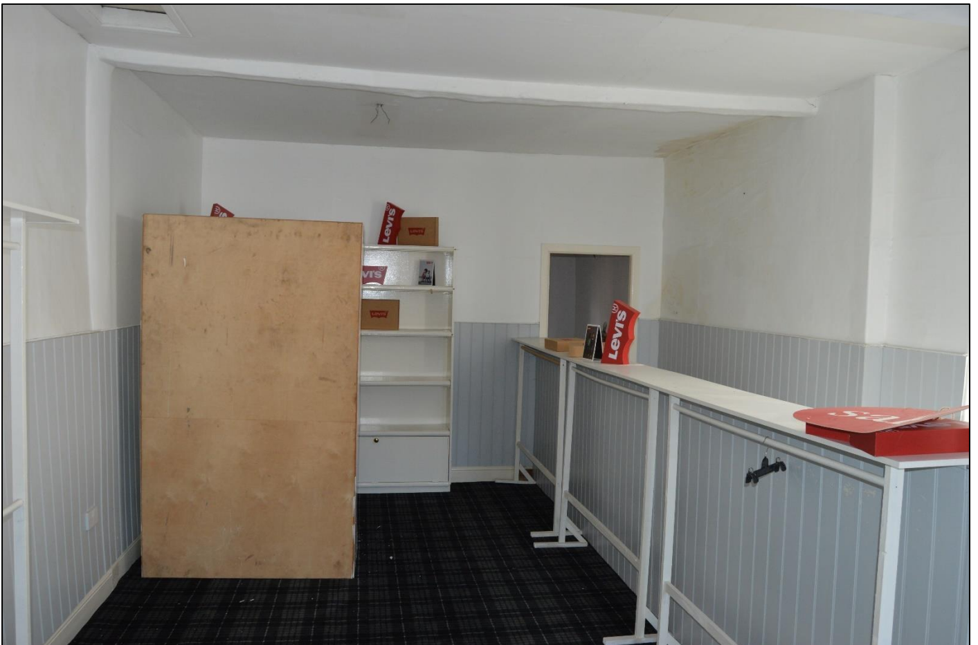
PL20: View northwest within the first-floor shop unit.
