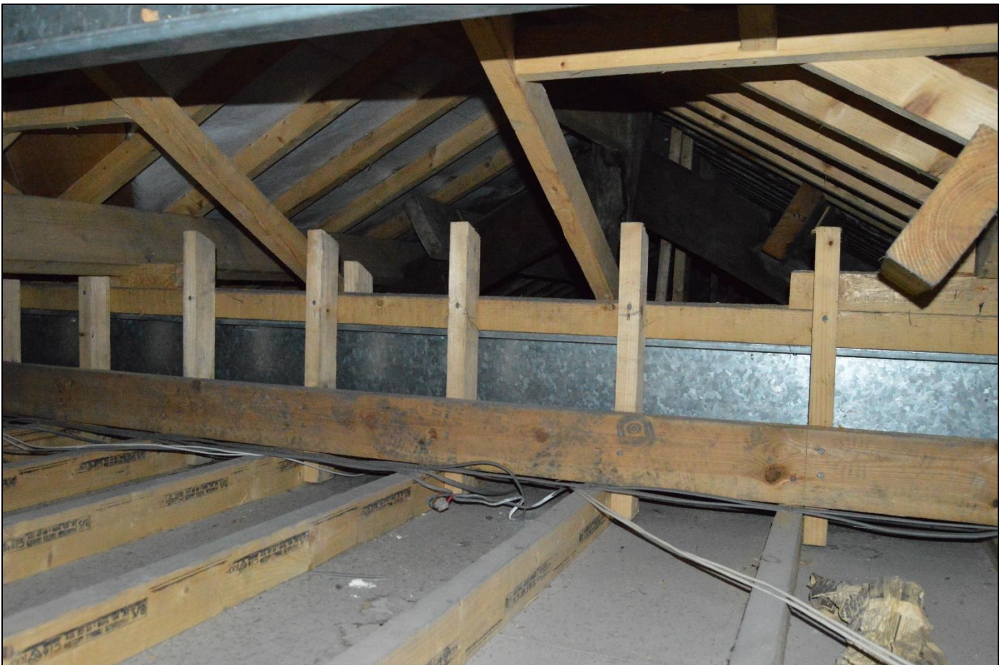
PL26: View of the roof structure over the southeast dual pitch roof, with the intersecting south east roof.
