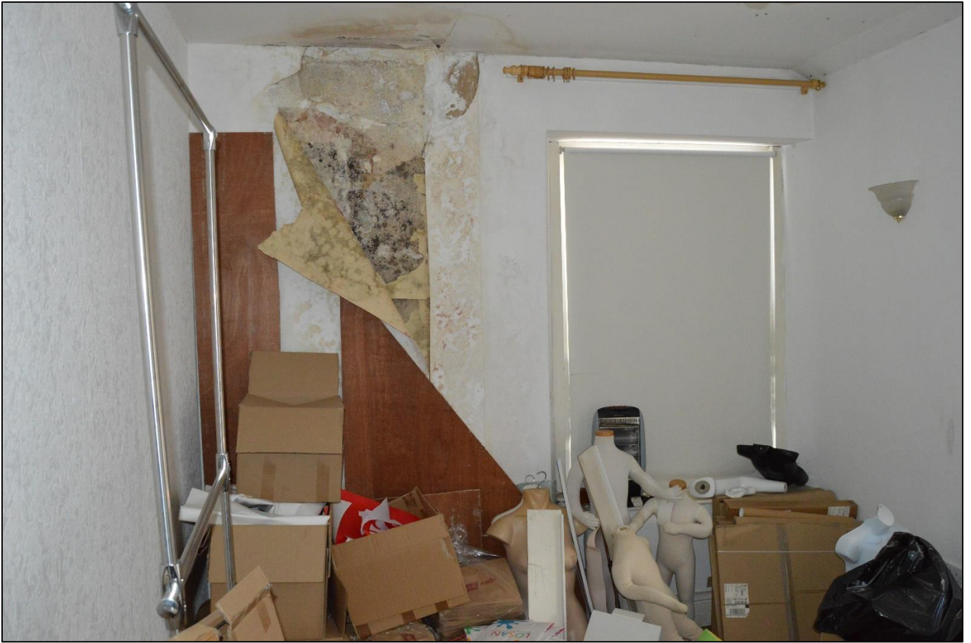
PL23: View southwest within the first-floor front unit.
