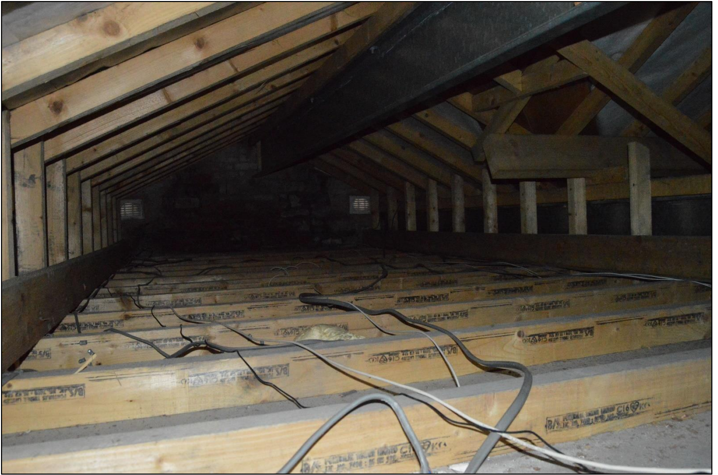
PL26: View of the roof structure over the southeast dual pitch roof.
