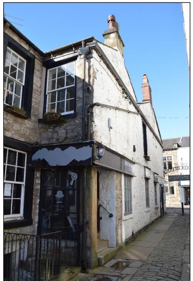
PL03: View of 26 Castle Street from the east.
