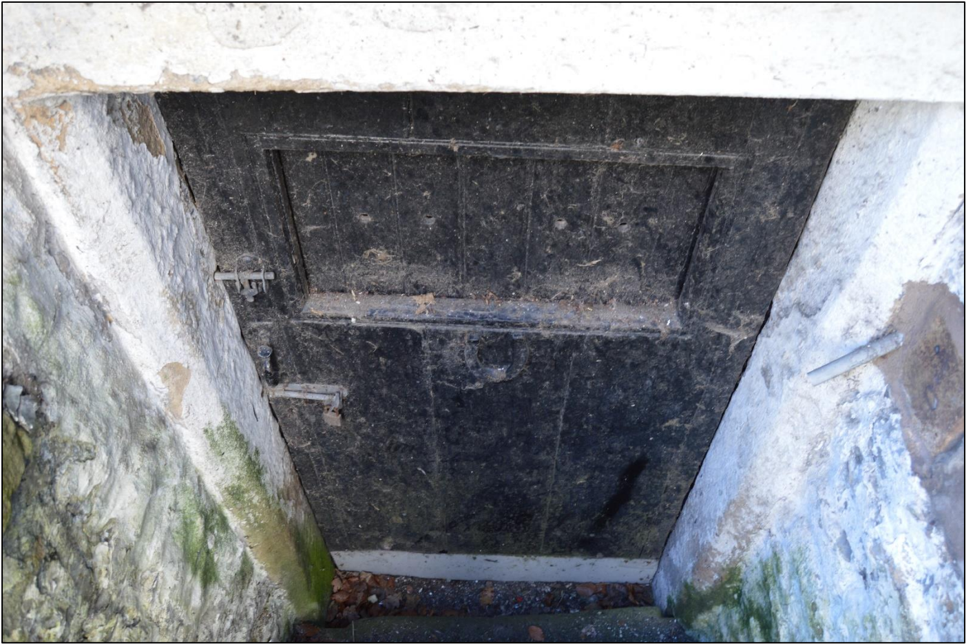
PL04: View of the 17 th century basement doorway to the northeast elevation.
