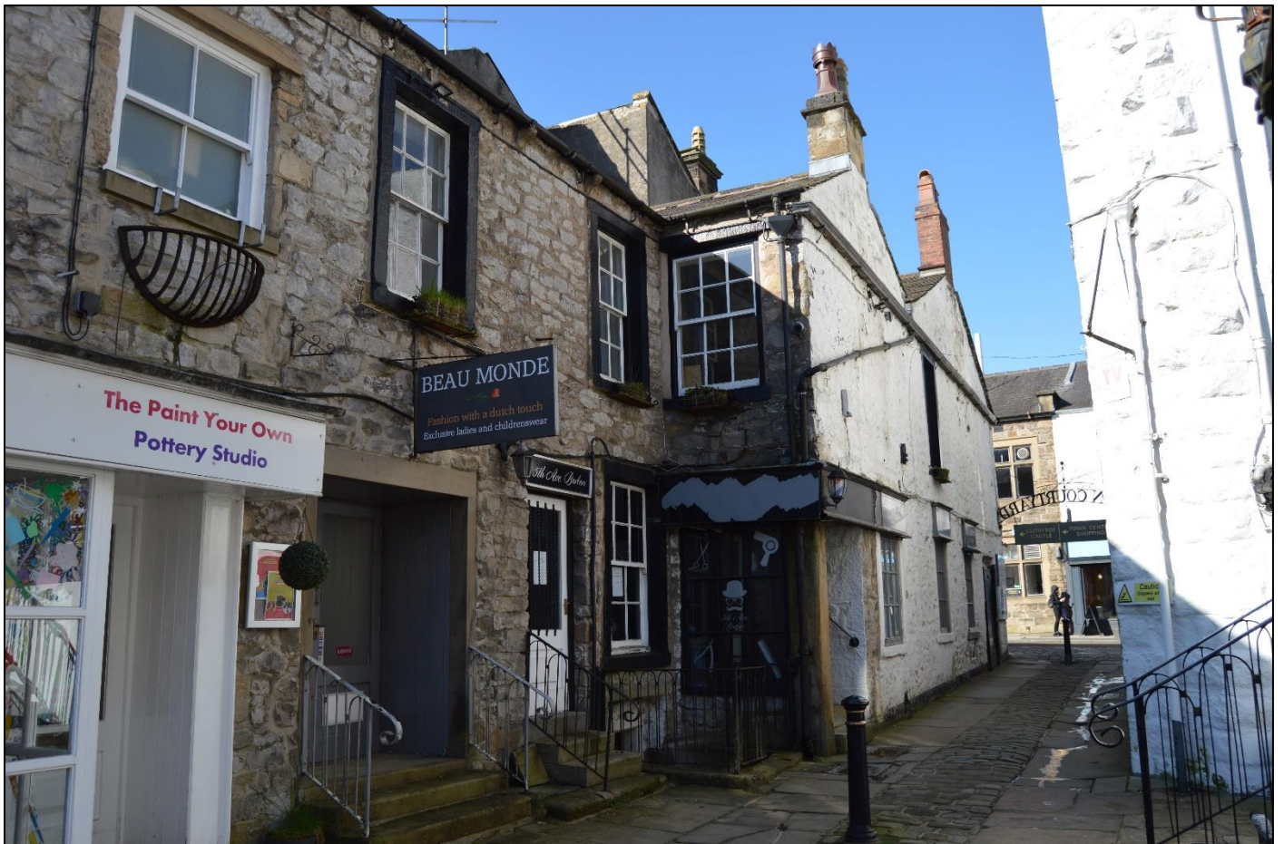
PL05: View of 26 Castle Street from the east.
