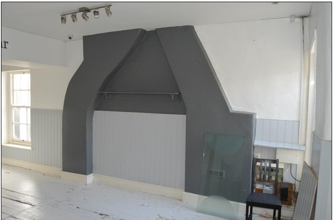
PL18: View of the chimney breasts to the first-floor shop unit.
