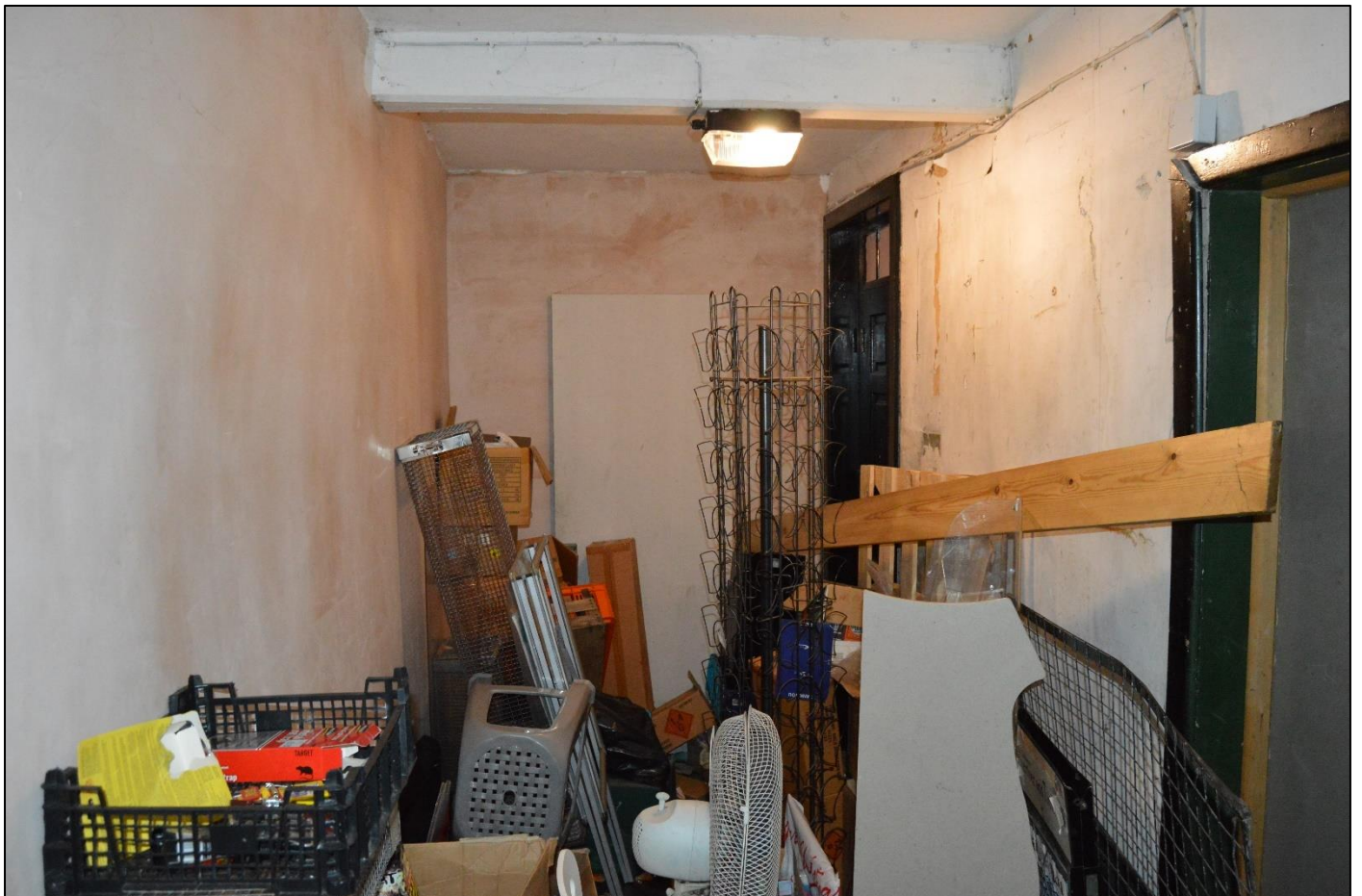
PL14: View northeast in the ground floor rear shop unit.
