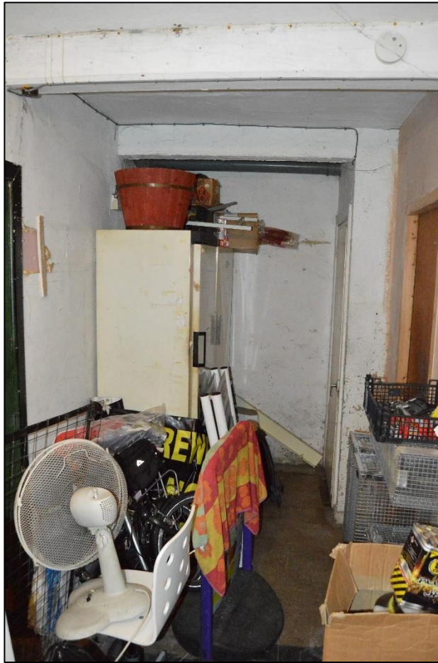
PL13: View southwest in the ground floor rear shop unit.
