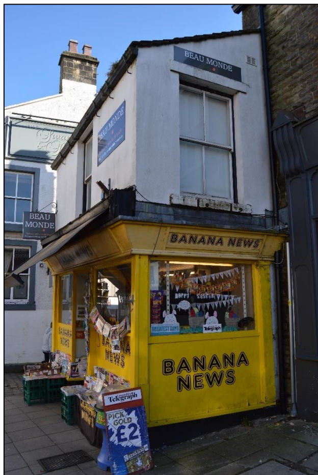
PL02: View of 26 Castle Street from the southeast.
