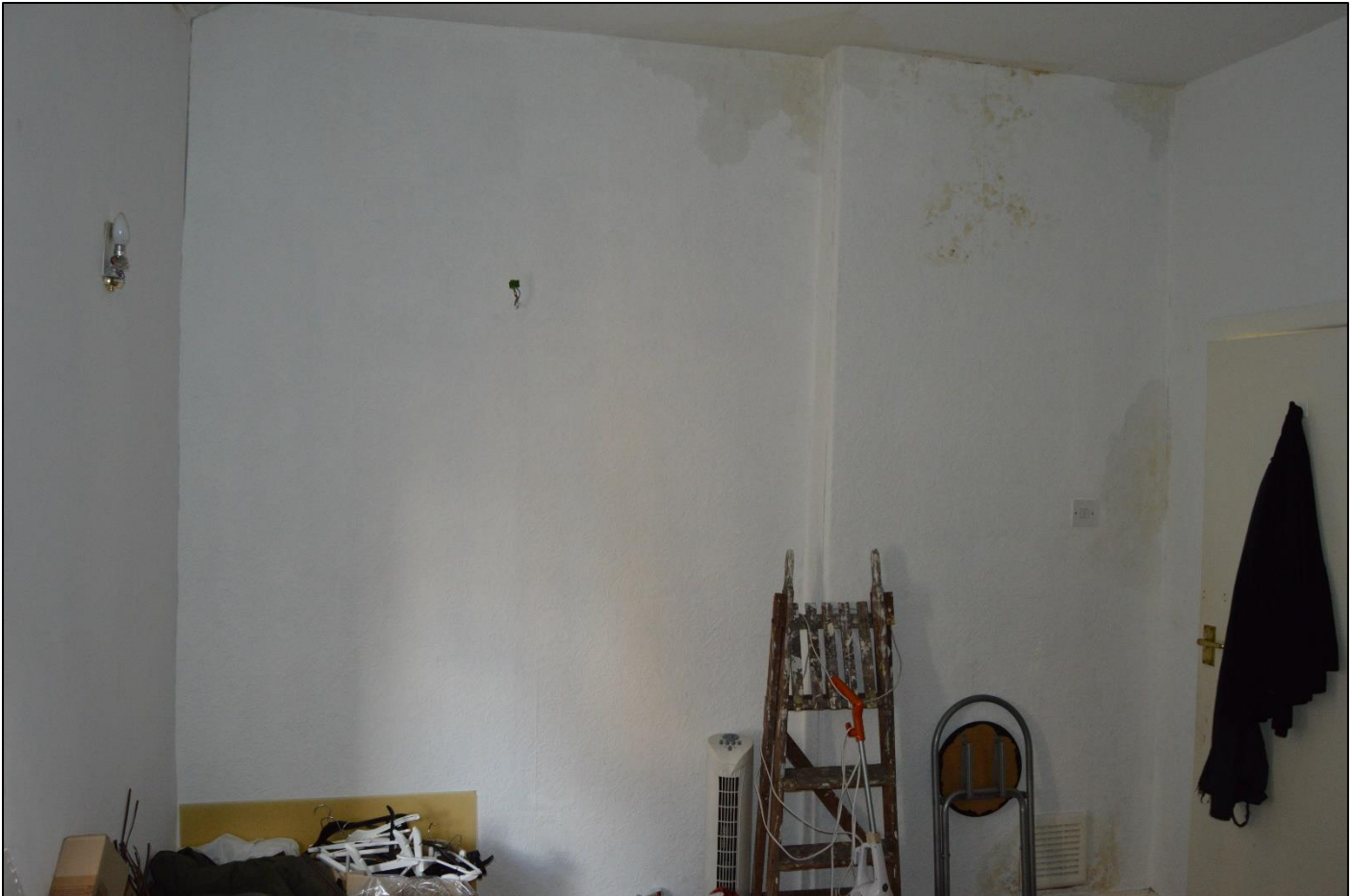
PL21: View northeast within the front first floor unit.
