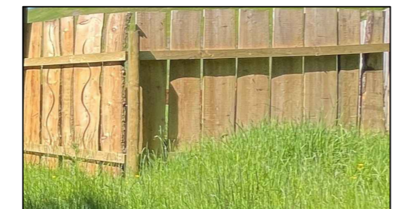
Picture of 1.7m Fencing
