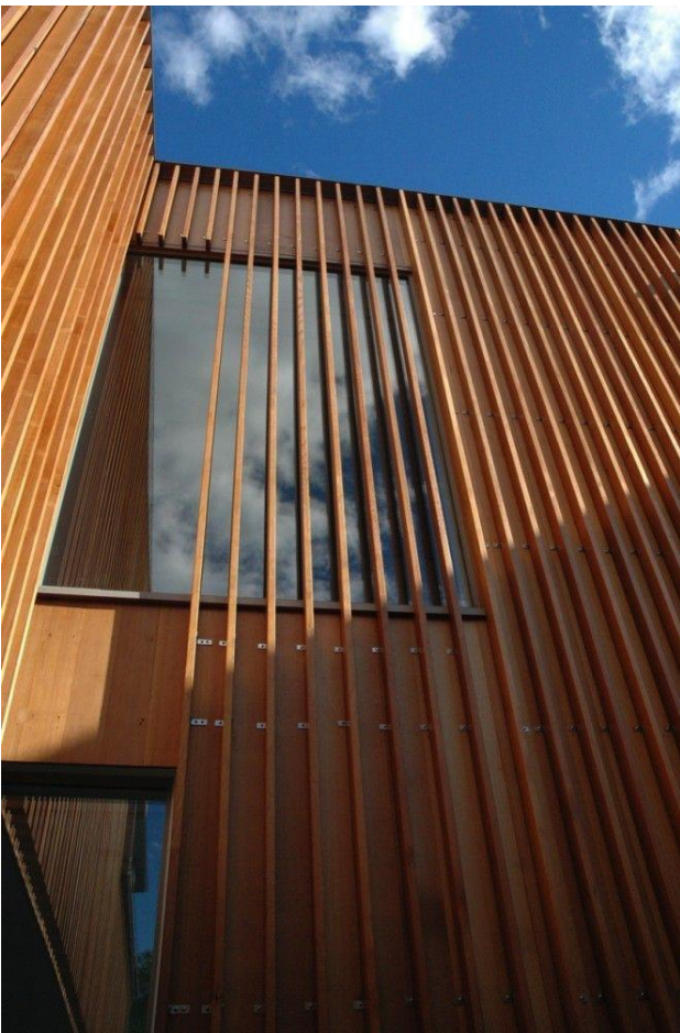
IMAGE SHOWING CLADDING OVER GLAZING TO LESSEN GLAZING IMPACT WHILST PROVIDING NATURAL LIGHT AND OUTLOOK
