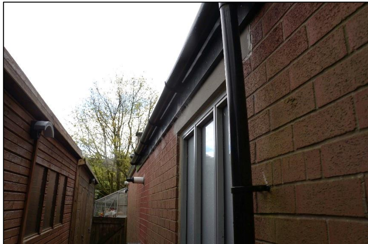
Photo 4: north elevation showing close-up of gutter and back board, all in a good state of repair.
