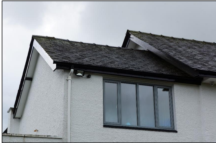
Photo 3: east elevation, showing roof tiles and ridge in good order.
