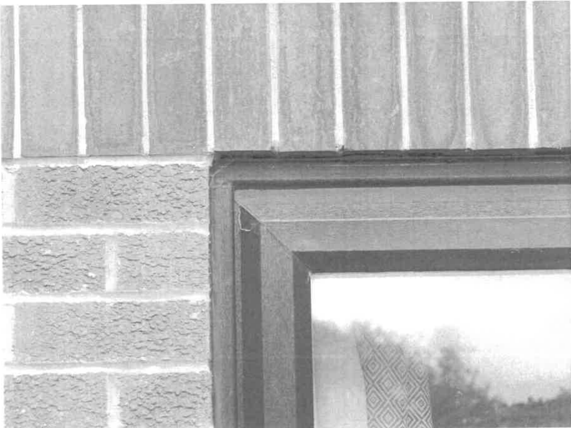
6 – Brickwork, mortar, and window frames are in good condition with no suitable gaps.
