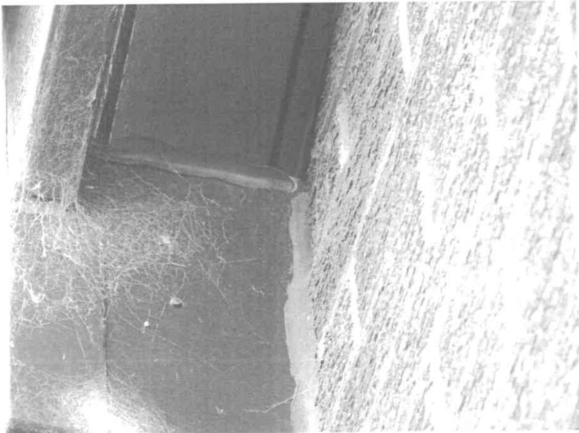
4 – Fascia boards and soffits at the eaves and gables are fixed tightly against brickwork.
