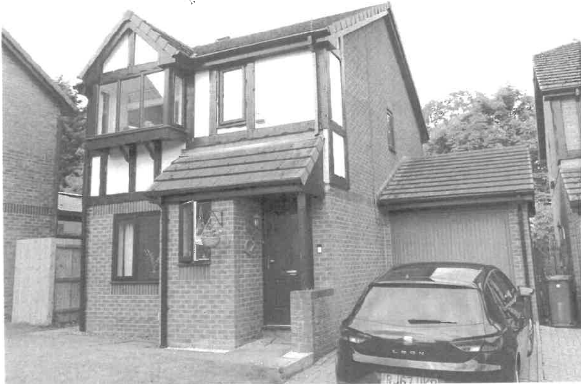
3.1a – The front of the house.
