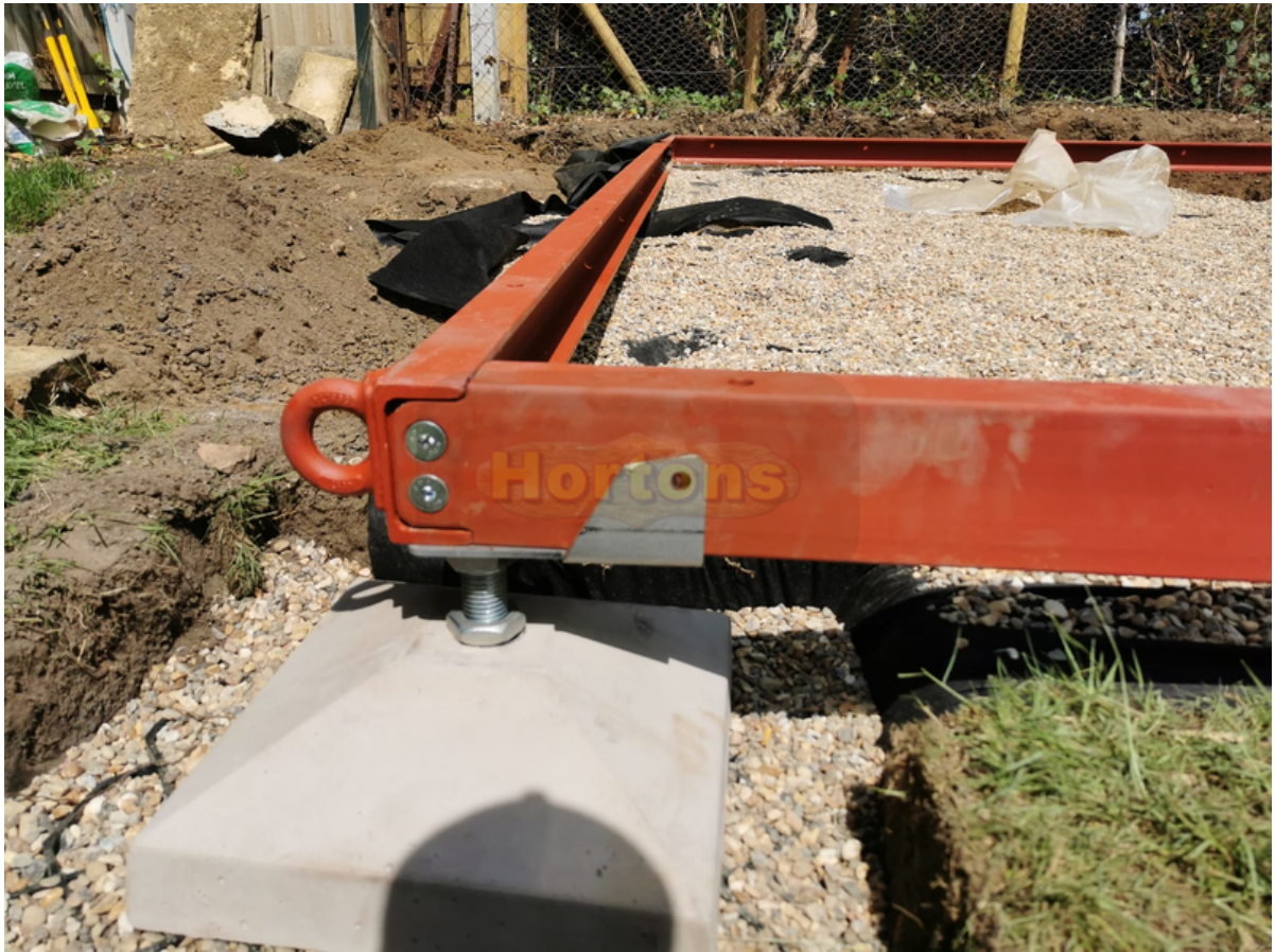
Illustration of proposed structural chassis construction including lifting eyes.
